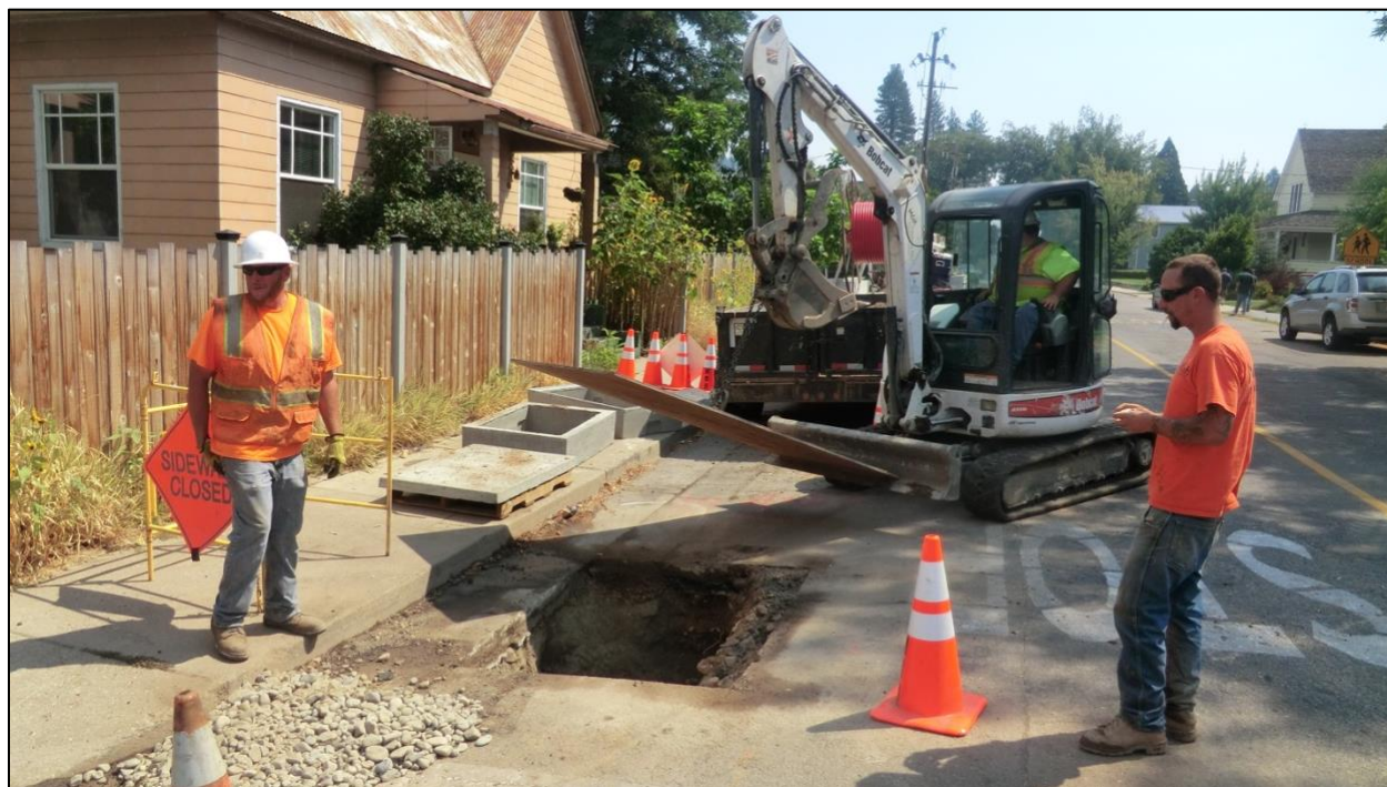
Figure 3 – Crews installing CPUC-funded fiber infrastructure in Quincy (Plumas County).
