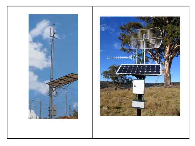
Capturing mobile reception: Grid Antenna connected by a cable to a broadband mobile modem connected by USB to a router connected by a cable to an antenna powered by Cow Shades using solar panels, a Regulator & Battery storage to power the unit at night and cloudy days.
