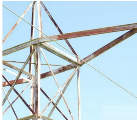
Paint Deteriorating
