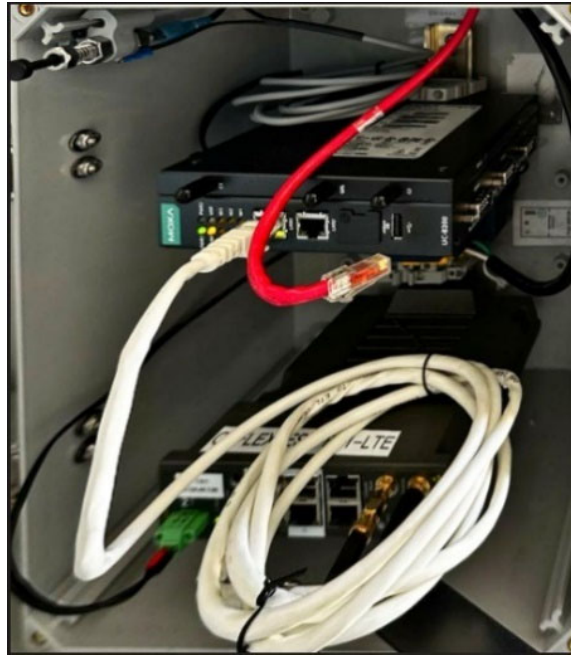
Figure 0-9. Modbus Gateway Disconnection from MBESS Local Controller to Emulate the Communication Loss Scenario
