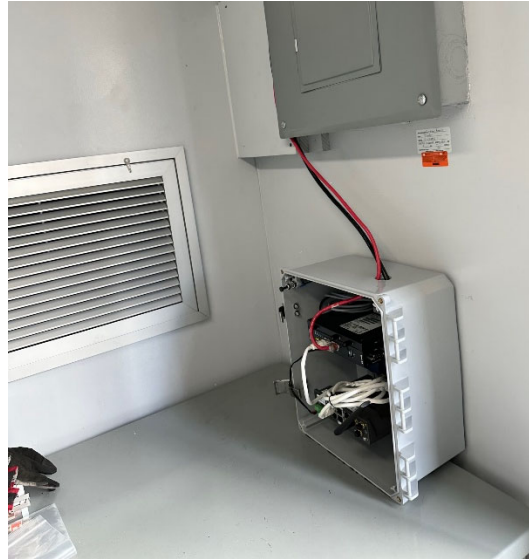
Figure 0-2. Gateway Installation for MBESS Integration with IEEE 2030.5 Standard
