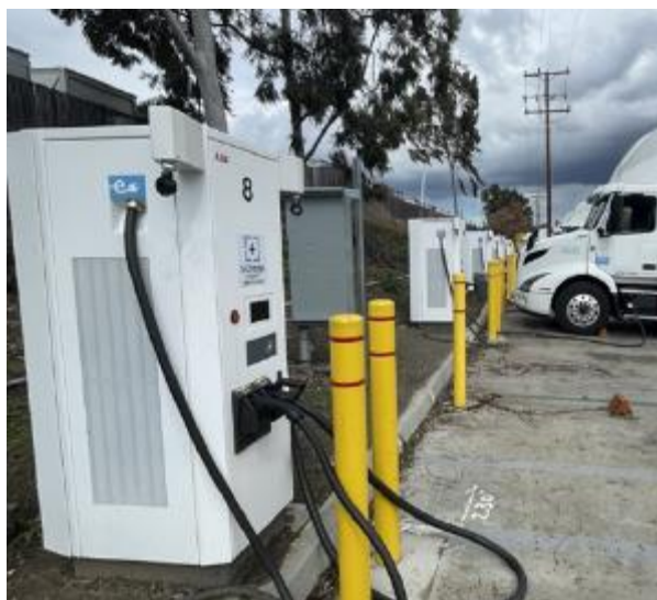
Figure 20. Heavy-Duty Charging in Softscape
