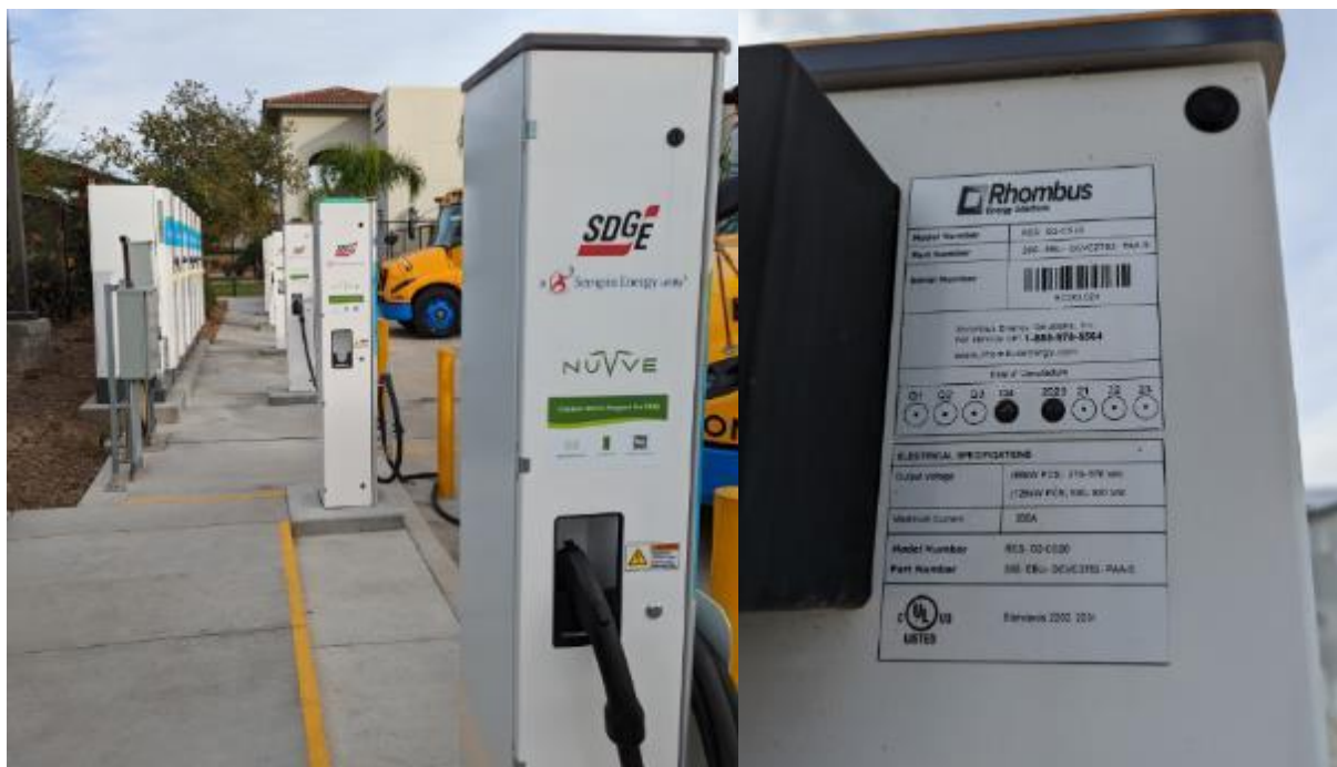
Figure 198. Nuve Rhombus DCFC Chargers (left: separate power cabinets and dispensers; right: Rhombus nameplate)
