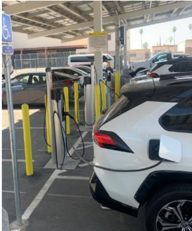
Figure 52. SCE Schools and Parks Pilot Head-to-Head Parking Resulting in Each Port Reaching 2.2 Spaces
