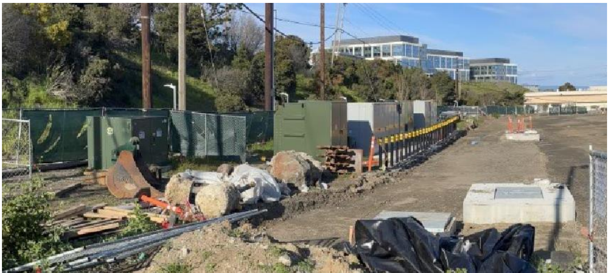
Figure 81. PG&E EV Fleet Program Inset of Above Photo Showing Transformers, Switch Gear, and Stub Outs
