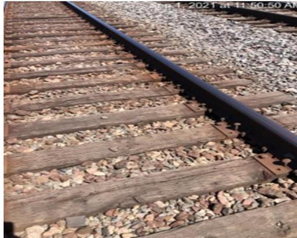
Track section with loose and missing fasteners
