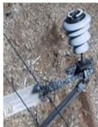
Figure 33: Loose tie wire (left) and resulting pole fire (right) 123
