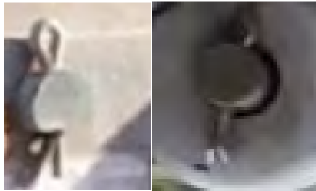
Figure 41: Examples of PG&E fully inserted cotter keys 186
