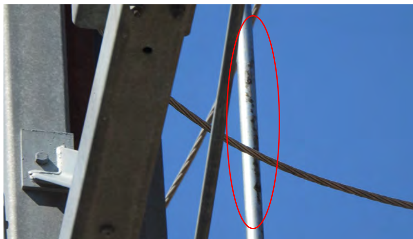
Figure 11: Control rod next to Switch 47 jumper. Red indicates damaged section of control rod. 41
