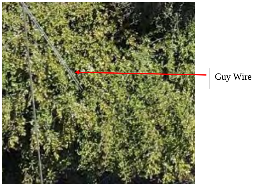
Figure 43: Vegetation obscuring guy wires at Pole 000/003 192
