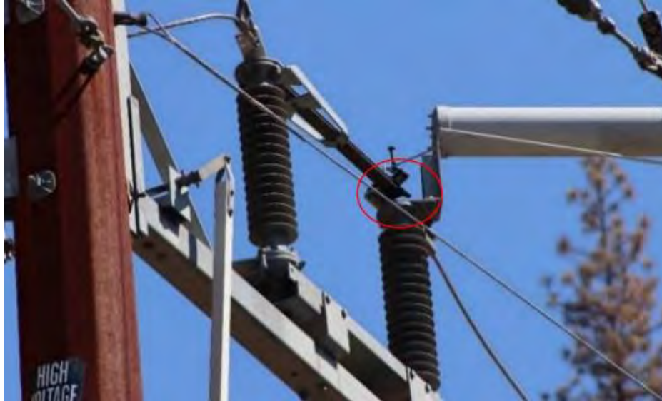
Figure 5: Switch 47 bottom phase in closed position. Red circle shows rotating end of blade within jaws. 34
