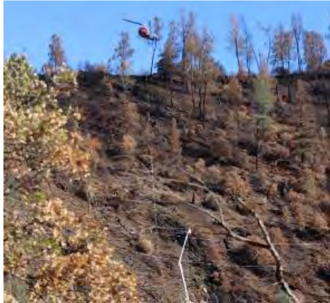
Figure 14: Conductor collection by helicopter and bucket truck 48
