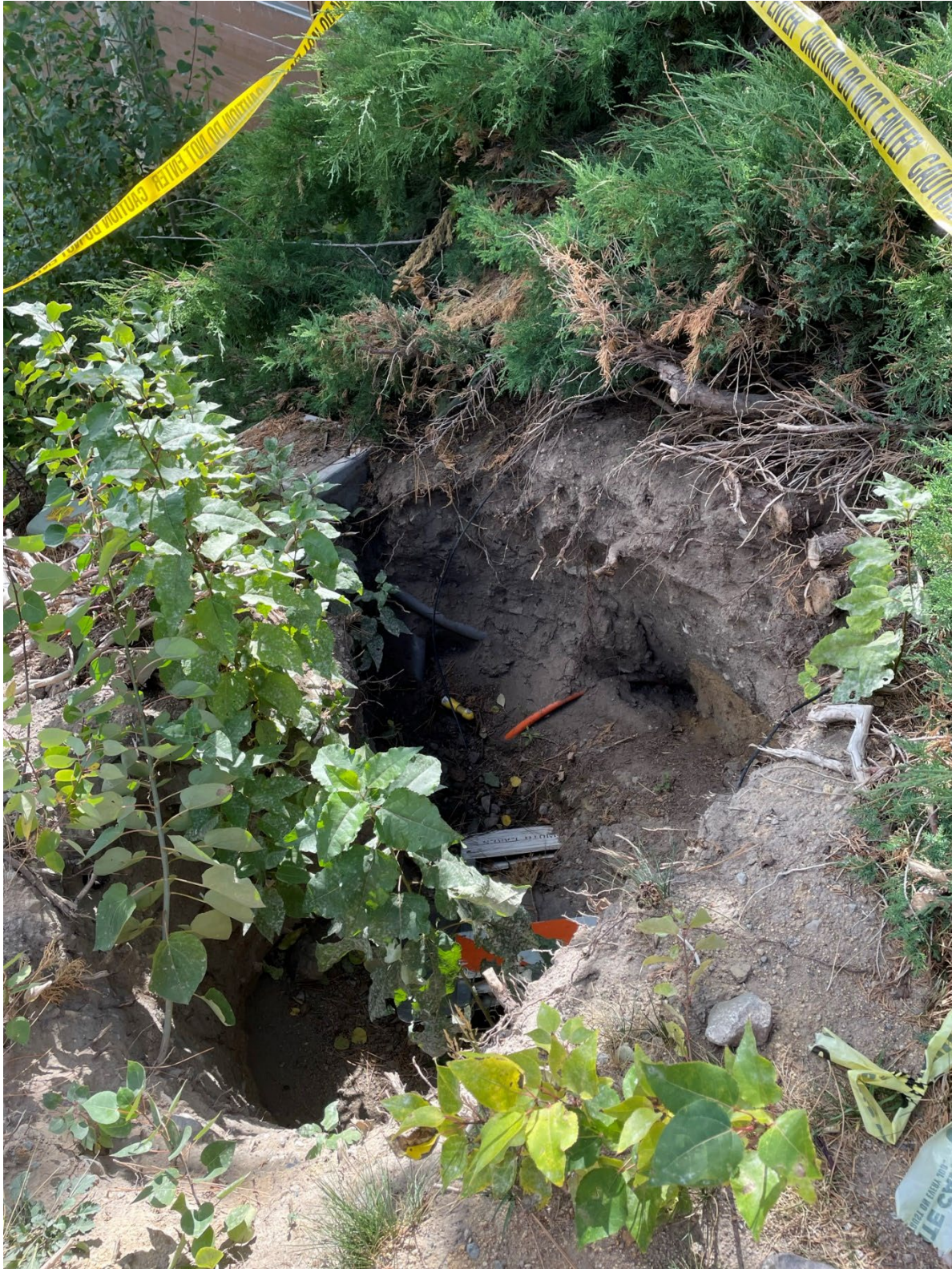
Figure 2. Excavation on southwest corner of property to locate and squeeze service line, taken from the west on 9/21/23.
