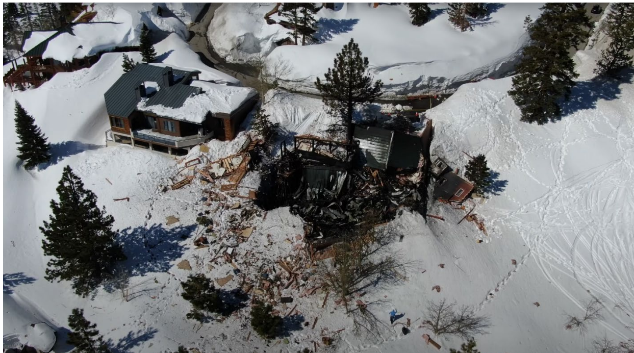
Figure 6. Aerial drone footage overview of incident site taken from the east on 4/2/23. Snow banks are taller than the fire engine (approximately 10-12 feet) just concealed on the top right portion of street.
