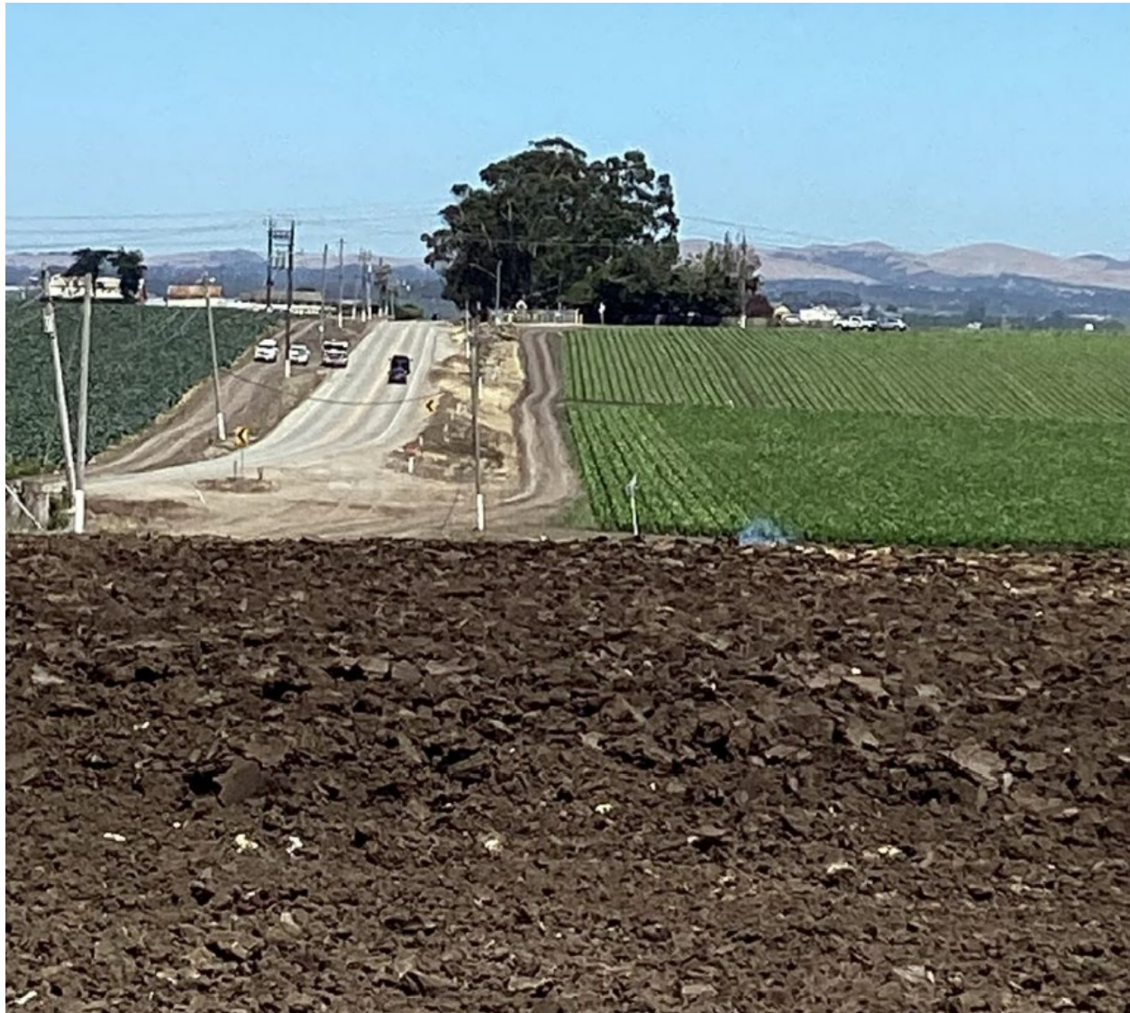
Figure 2. Photo from the incident location, following the line to a valve station. Note the pipeline marker, and missing USA markings on the ground.
