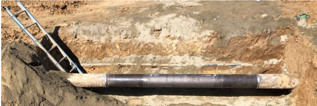
Figure 3. New section of 10-inch HPDSM pipe; replaced steel pipe with permanent repair
