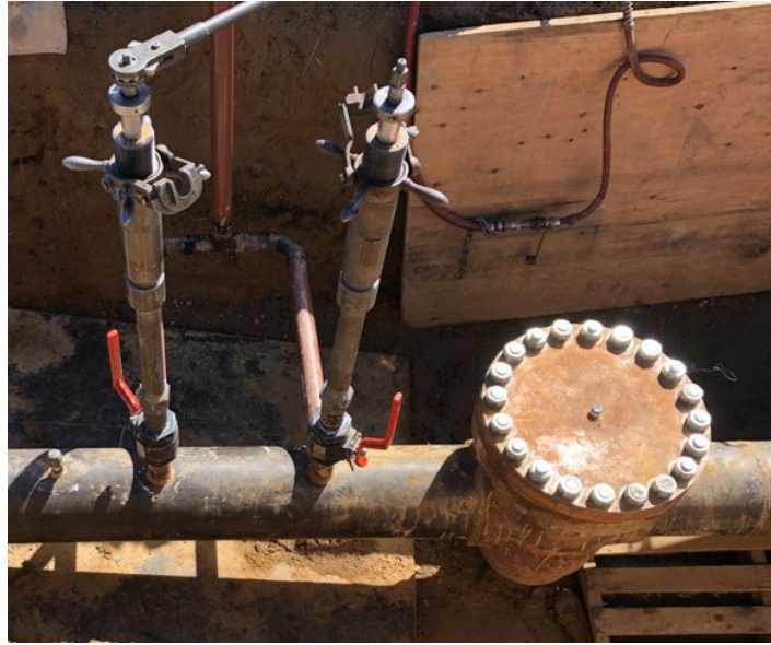
Figure 1. Pressure control fittings and stopper
