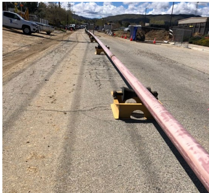
Figure 2. Temporary bypass pipeline
