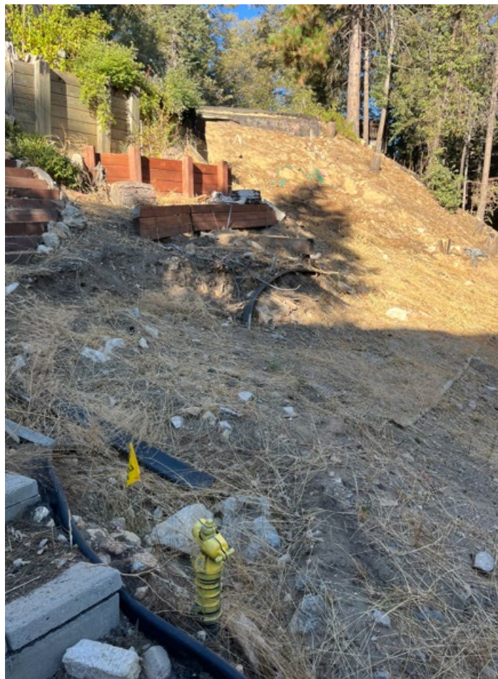
Figure 3. SoCalGas removed MSA from service and locked service riser at [REDACTED] Augusta Drive, Lake Arrowhead
