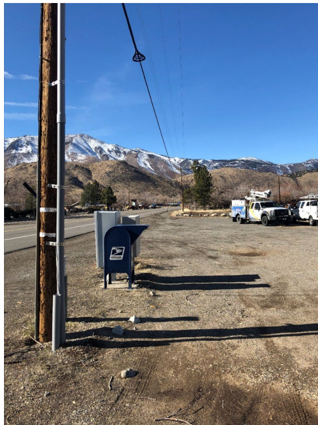
Figure 2: Repaired span at the incident location 2
