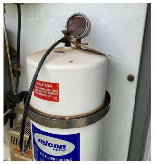
We agree a transformer oil filter was reaching its replacement threshold at Sisquoc Sub. This nonconformance has a pre-existing notification 127576246 established in our system of record SAP prior to the field audit. We do not agree that this finding qualifies as a violation of GO 174, Rule 12 since this notification was being worked in accordance with our maintenance procedures and was completed on December 13, 2024.
