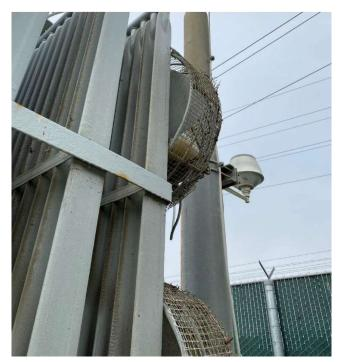
4.2. The top cooling fan on Transformer 21 could not start automatically and required manual assistance to start rotating. Additionally, there are large gaps in the fan blade covers that can expose workers to hazards. PG&E immediately created the Notification #129692075 to address the issue.
