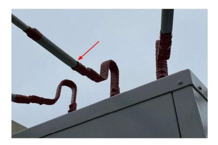
We agree with the finding of the exposed bus conductor due to a gap in the animal abatement on 1102/2 at Cayucos Substation. We created notification 130717744, which will be completed based on current work prioritization and material availability.
