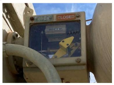
We agree a faded counter was present on CB 152 at Sisquoc Sub. This nonconformance has a pre-existing notification 125554093 established in our system of record SAP prior to the field audit. We do not agree that this finding qualifies as a violation of GO 174, Rule 12 since this notification was being worked in accordance with our maintenance procedures and was not past due. However, this work was completed on December 2, 2024.
