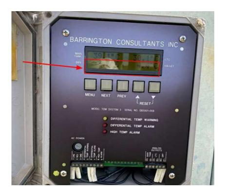
We agree with the finding of the impacted display on the Barrington LCD screen at Zaca Substation. We created notification 130717745, which will be completed based on current work prioritization and material availability.
