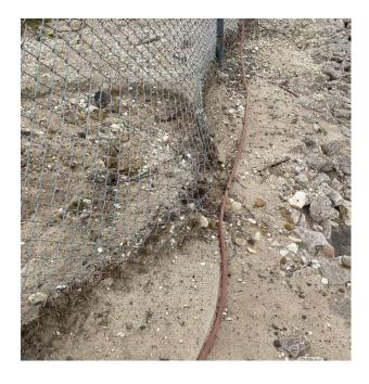
PG&E Response: We agree erosion and washout was present at the perimeter fence at Palmer Sub. This
