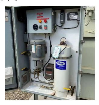
We agree the LTC Oil Filter Pump was out of service due to a leak was present at Buellton Sub. This nonconformance has a pre-existing notification 124791416 established in our system of record SAP prior to the field audit. We do not agree that this finding qualifies as a violation of GO 174, Rule 12 since this notification is being worked in accordance with our maintenance procedures and is not past due.
