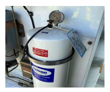
We agree with the finding of the LTC oil filter needing changing at Zaca Substation. We created notification 129771711, which will be completed based on current work prioritization and material availability.
