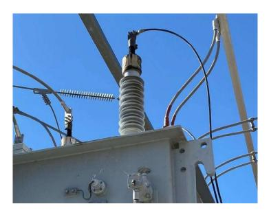
We agree one bushing on Transformer 1 is damaged at Atascadero Sub. This nonconformance has a pre-existing notification 128243310 established in our system of record SAP prior to the field audit. We do not agree that this finding qualifies as a violation of GO 174, Rule 12 since this notification was being worked in accordance with our maintenance procedures and was not past due. However, this work was completed on December 3, 2024.
