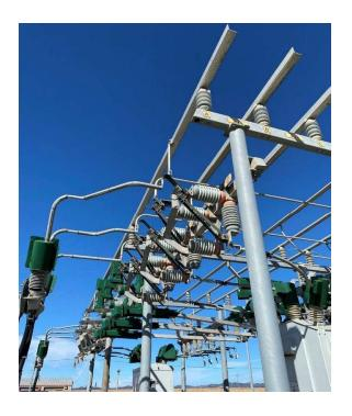
We agree with the finding of the loose bracket at the BUS support on 12kv Bus 2A at Cabrillo Substation. We created notification 130717748, which will be completed based on current work prioritization and material availability.
