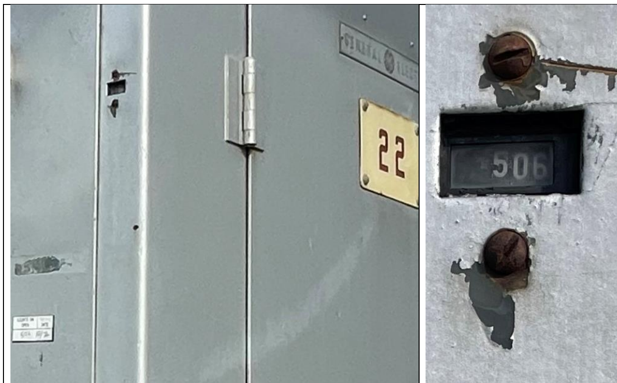
16.11. Circuit Breaker 42 has a damaged counter. PG&E indicated it has an existing LC notification for this issue: # 130881869.
