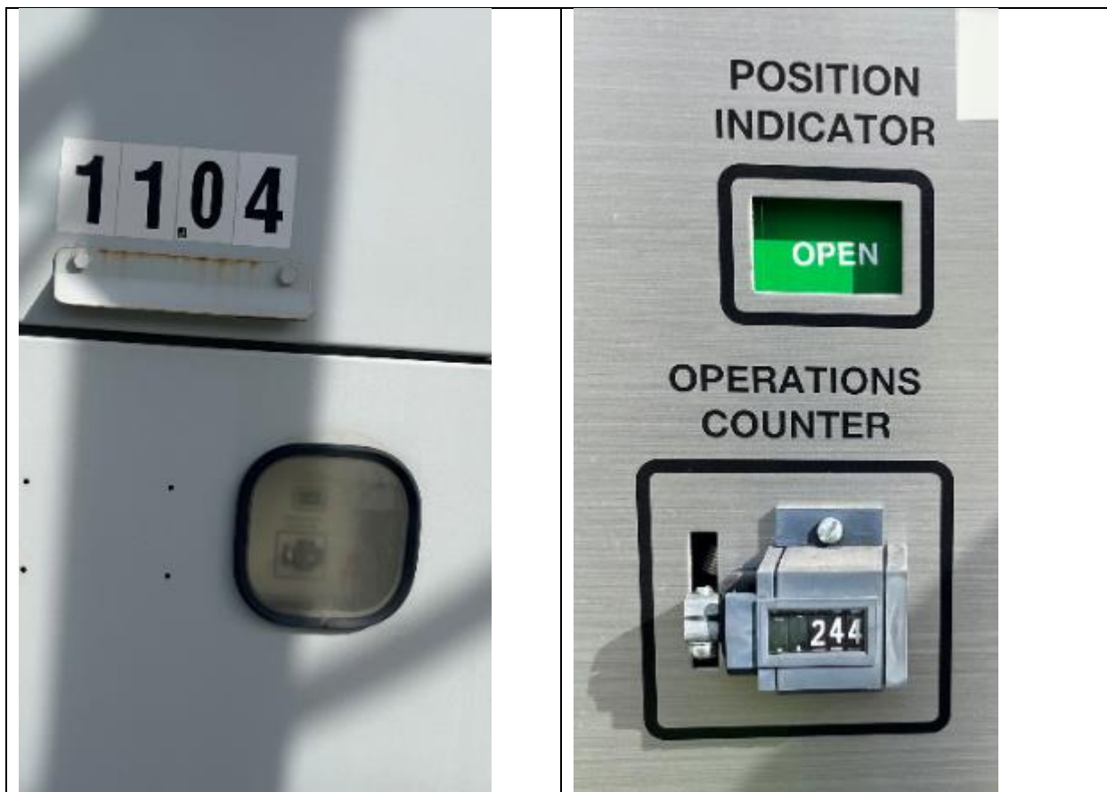
17.14 Circuit breaker 162 has a faded semaphore for the closed position.
