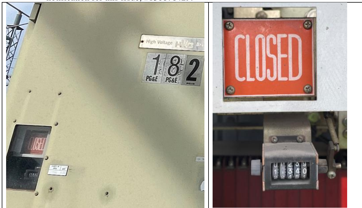
16.3. Circuit breaker 182 has a damaged counter. PG&E indicated it has an existing LC notification for this issue, #130876429.
