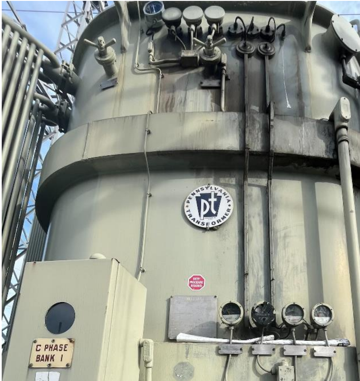
16.8. Transformer bank 1C has an oil leak.
