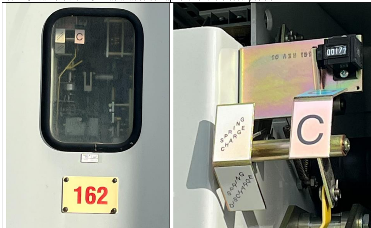
17.14 Circuit breaker 162 has a faded semaphore for the closed position.
