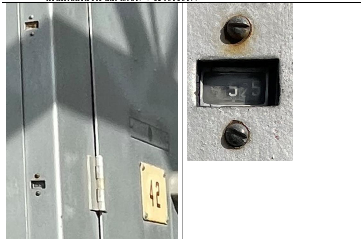
16.11. Circuit Breaker 42 has a damaged counter. PG&E indicated it has an existing LC notification for this issue: # 130881869.
