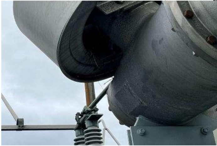
11.2 Circuit Breaker 112 Two Birds Nests, No Existing Tag Created New LC Tag#131982951
