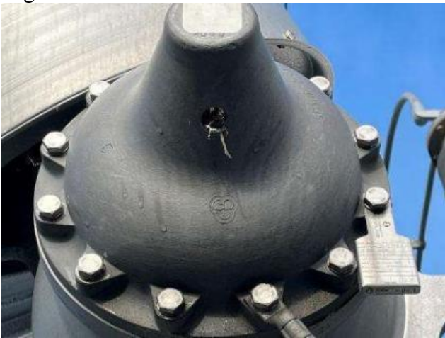
15.3 Circuit Breaker 72 Birds Nest Existing LC Tag#131964230
