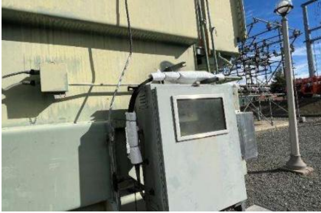
9.12 Transformer Bank 5 Nitrogen System Repair Possible Minor Leak Existing LC Tag#131966342 (Came and Replaced Tubing Where Leak Was & Now Monitoring)
