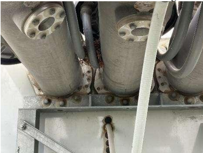
15.3 Circuit Breaker 72 Birds Nest Existing LC Tag#131964230
