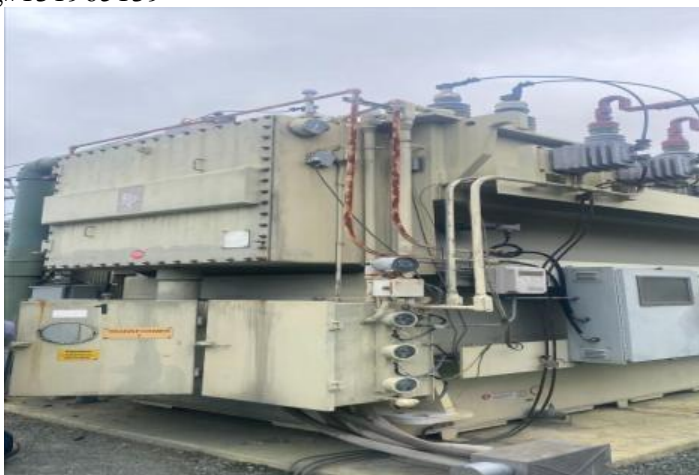
11.4 Transformer Bank 1 Oil Mitigation Leak Repair and Residue Cleanup Existing LC Tag#131965139
