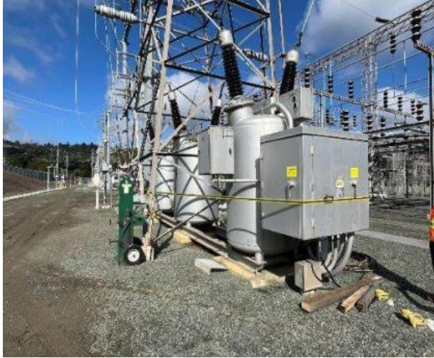
13.4 Circuit Breaker 1100 Faded Semaphore Will Add Sticker - Fixed in Field
