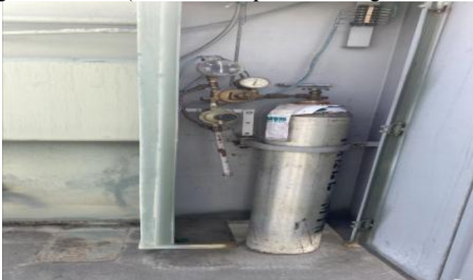
9.12 Transformer Bank 5 Nitrogen System Repair Possible Minor Leak Existing LC Tag#131966342 (Came and Replaced Tubing Where Leak Was & Now Monitoring)
