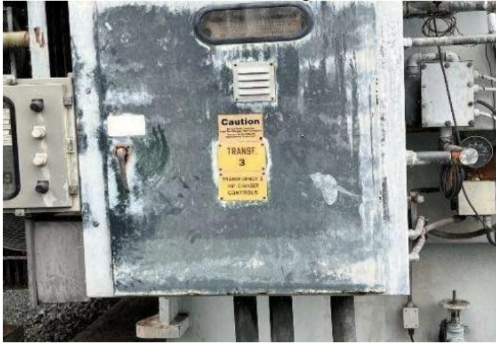
11.6 Transformer Bank 3 Oil Mitigation Residue Clean Up Existing LC Tag#131980352
