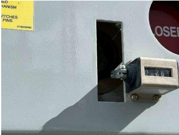
13.2 Circuit Breaker 372 Faded Counter, No Existing Tag, Created New LC Tag#131986539
