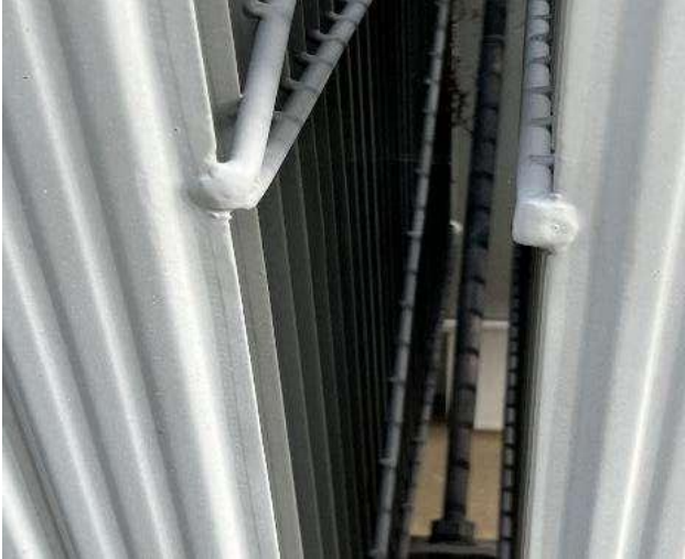
15.5 Transformer Bank 1 B Phase Oil Mitigation Existing LC Tag#131990028
