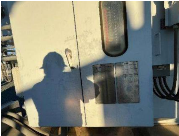
4.4 Observation: Transformer Bank 2 Missing Label For Target Plate Bank Number – Fixed In Field
