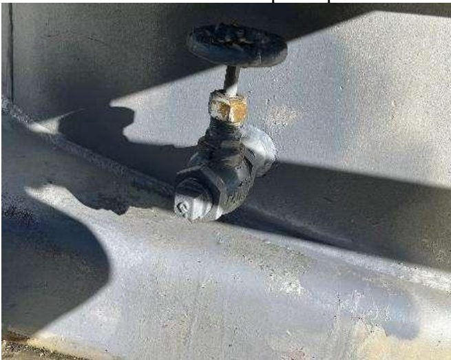
2.4 Transformer Bank 1C Oil Weep Sample Valve Nut Existing LC Tag #131971833
