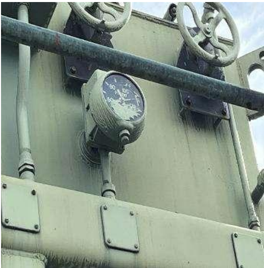
5.7 Transformer Banks 1A, 1B, 1C Thermal Load Gauges Not Working (Gauge Below Horizontal Green Scaffolding). PG&E plans to fix the issue in Capital Project 74066965 - Transformer Bank 1 Reseal All Phases and Replace Bushings
