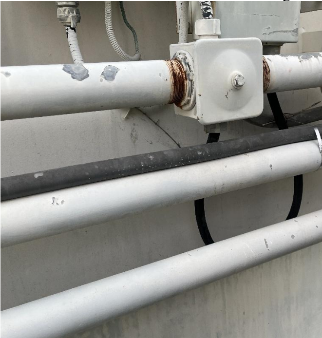
9.6 Transformer Bank 3 Birds Nest Near Nitrogen Bottle – Fixed In Field
