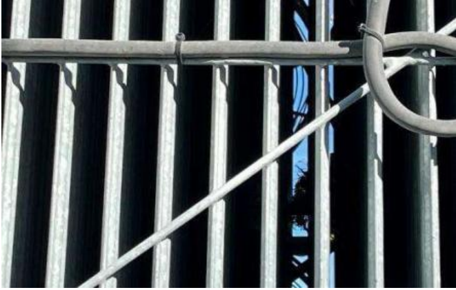
5.16 Voltage Regulator 3 (Currently Out Of Service) Oil Leak Mitigation Existing LC Tag#131966022, Needs Target (Name) Plate Label, Dissolved Gas Analysis Monitor to be Installed as Part of Capital Project
