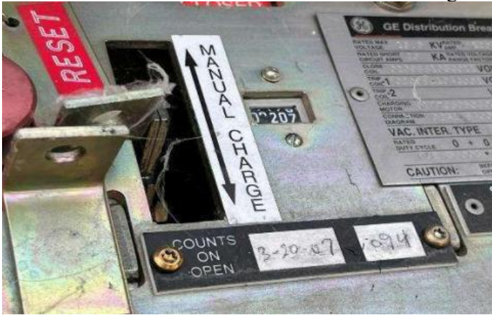
6.8 Perimeter Fence Missing Ground Rod on Corner Post New LC Tag#131977807
