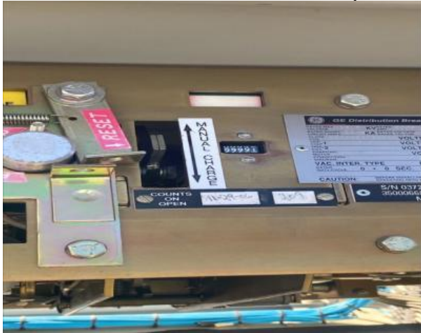
13.4 Circuit Breaker 1100 Faded Semaphore Will Add Sticker - Fixed in Field
