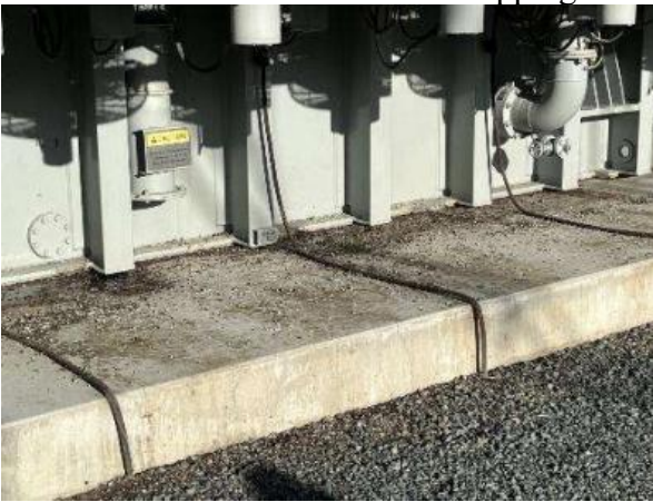
14.9 Voltage Regulator 1 Oil Leak Mitigation Existing LC Tag#131966575, Birds Nest LC Tag#131966574, Will Be Replaced with Transformer Bank 1 Capital Job
