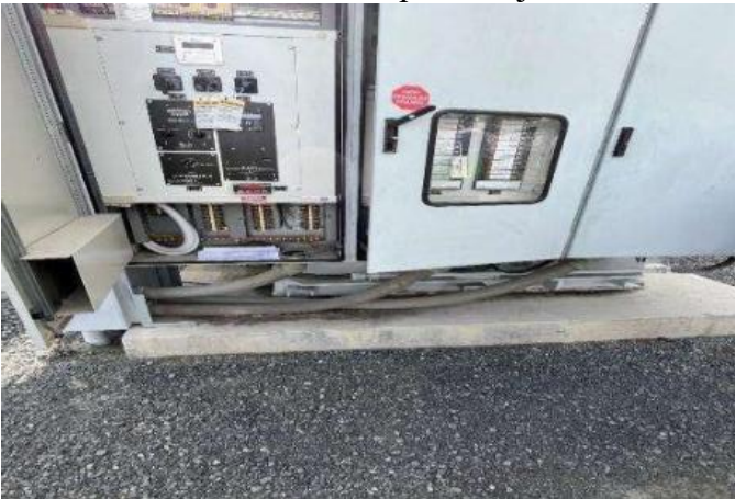
5.16 Voltage Regulator 3 (Currently Out Of Service) Oil Leak Mitigation Existing LC Tag#131966022, Needs Target (Name) Plate Label, Dissolved Gas Analysis Monitor to be Installed as Part of Capital Project
