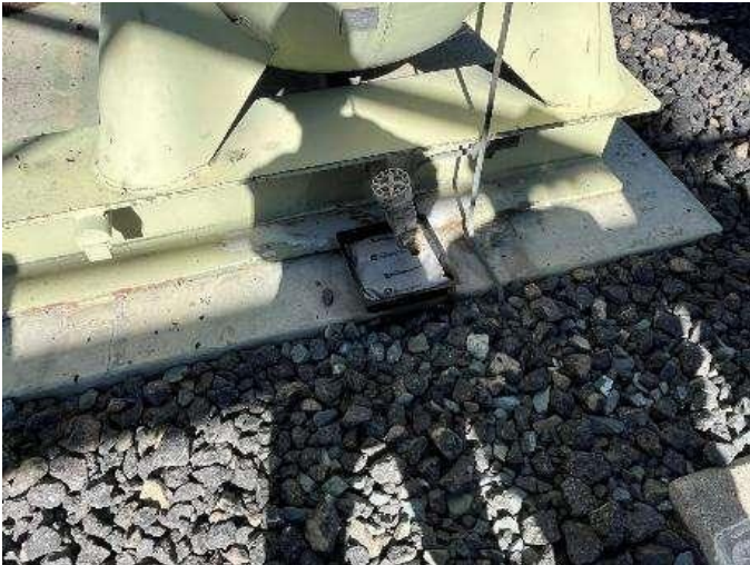
1.5 Circuit Breaker 570 (Out Of Service) Reservoir C Sample Valve Oil Leak Existing LC Tag#131965864
