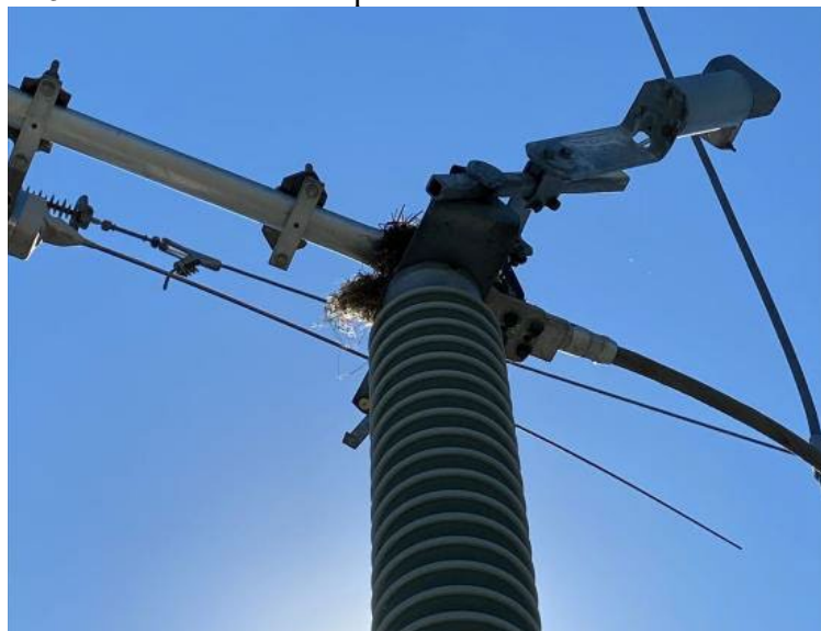
19.2.Switch 125 has a bird nest in C phase.
