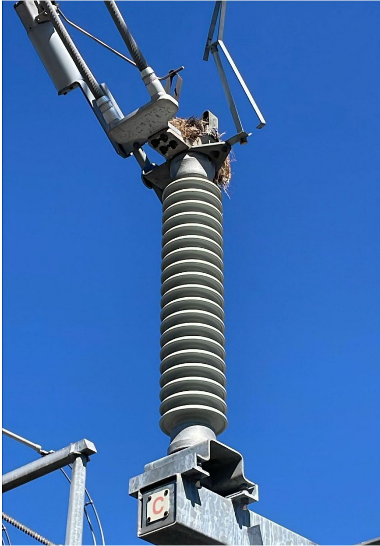
19.2.Switch 125 has a bird nest in C phase.
