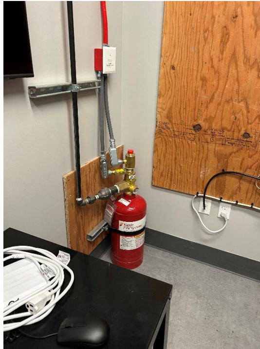
Figure 2: NOVEC system found in server room.
