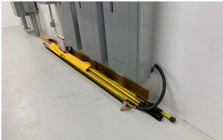
Figure 1: Outdated hot sticks left in the substation control house.
