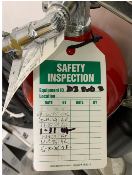
Figure 7: Fire extinguisher with missing monthly inspections.
