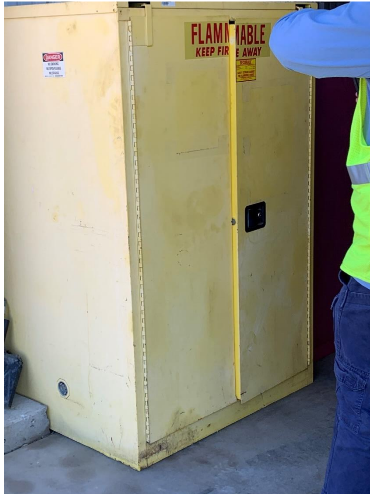
Figure 6. Flammable material storage cabinet [REDACTED] after letting the door attempt to close freely.
