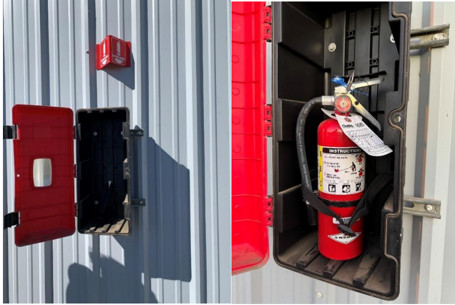
Figure 1: Missing (Left) and Replaced (Right) fire extinguisher [REDACTED]
