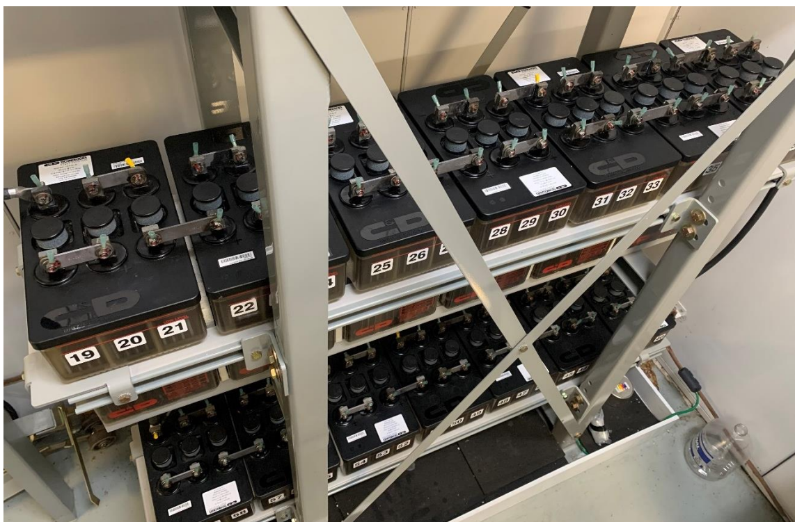
Figure 8: Battery rack after cleaning the terminals
