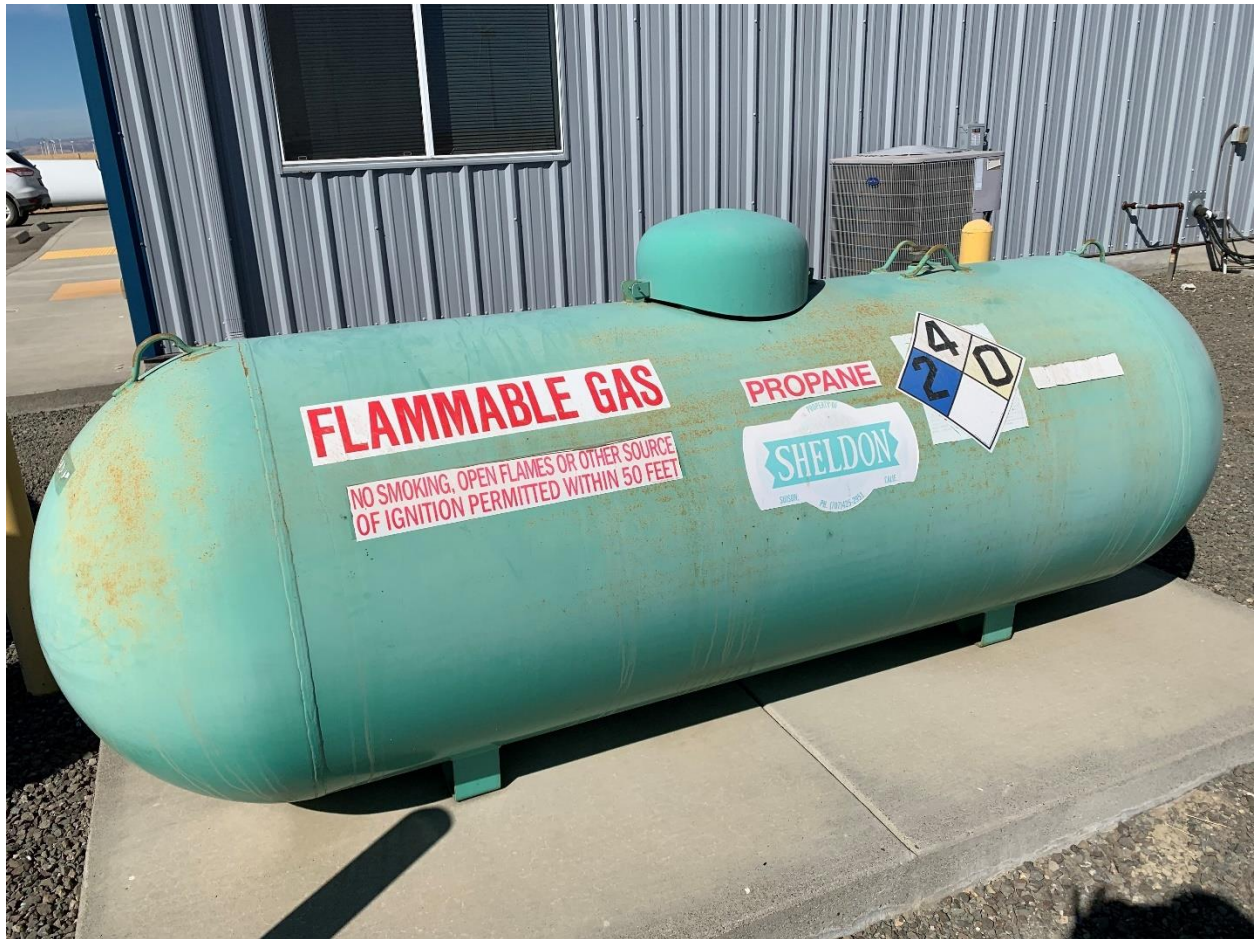
Figure 3: NFPA 704 placard on propane tank [REDACTED] s faded.
