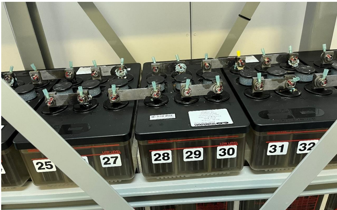
Figure 7: Battery rack with corrosion on terminals.
