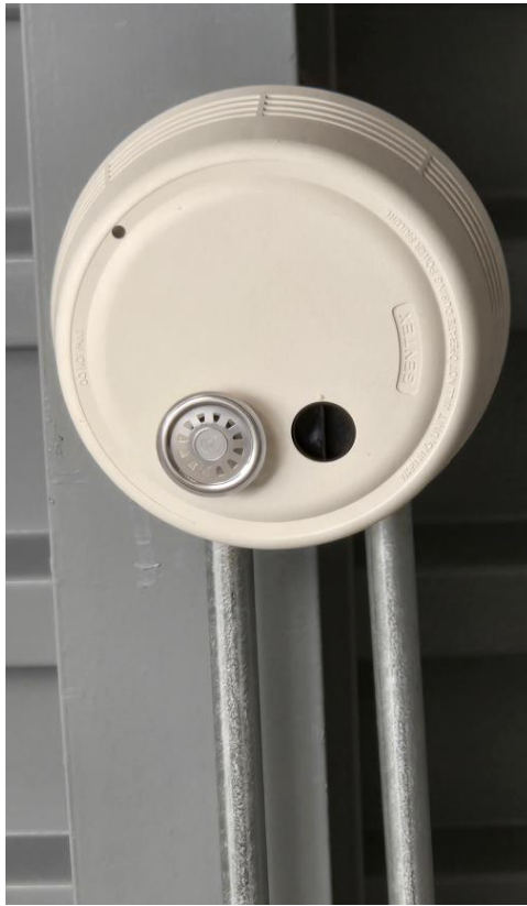
Figure 1: Battery room exhaust fan sensor with no method for functional testing.
