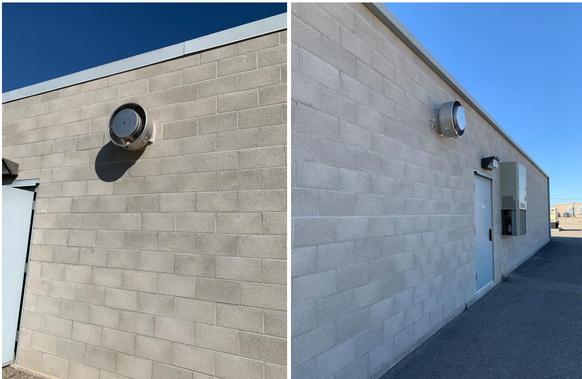
Figure 2: North and south-side exhaust fans lack a method for functional testing.
