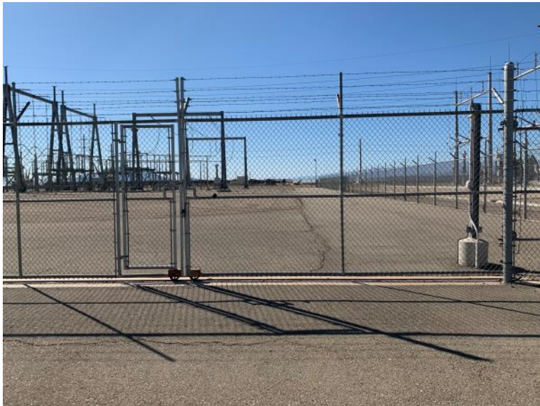
Figure 4: Dunaway switchyard front gate with missing NFPA 704 placard and high voltage signage.
