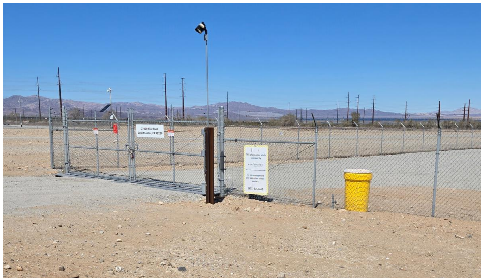
Figure 3: Oberon 1 BESS yard gates missing an NFPA hazard placard.
