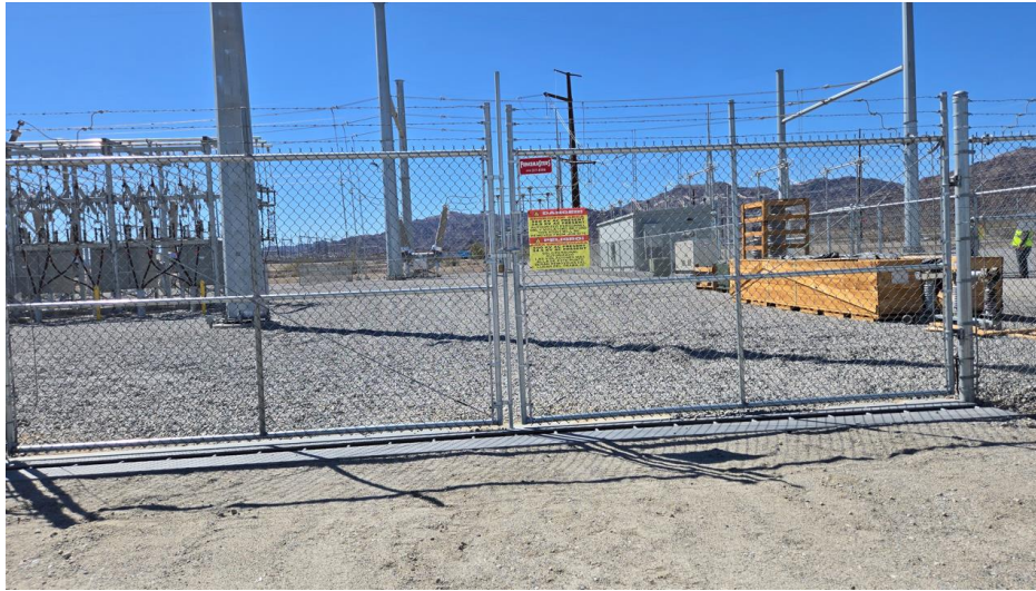
Figure 2: Substation gates missing an NFPA hazard placard.
