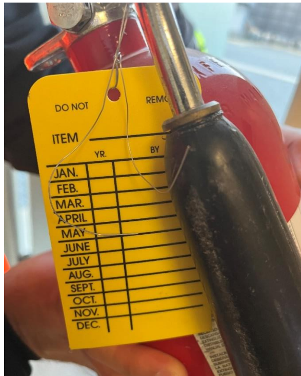
Figure 5: Blank Monthly Inspection Tag
