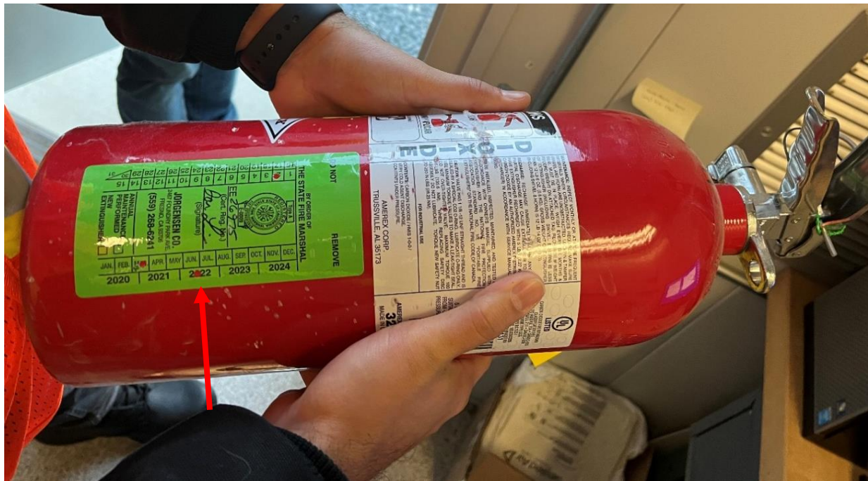
Figure 6: Fire extinguishers last inspected in 2022.
