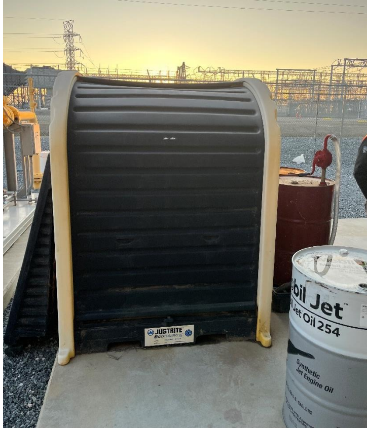
Figure 15: Containment bin missing NFPA 704 placard.
