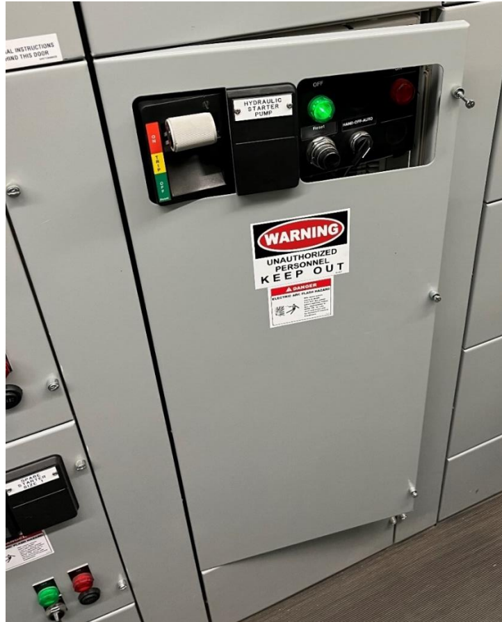
Figure 1: Unattended Hydraulic Starter Pump Cabinet ajar
