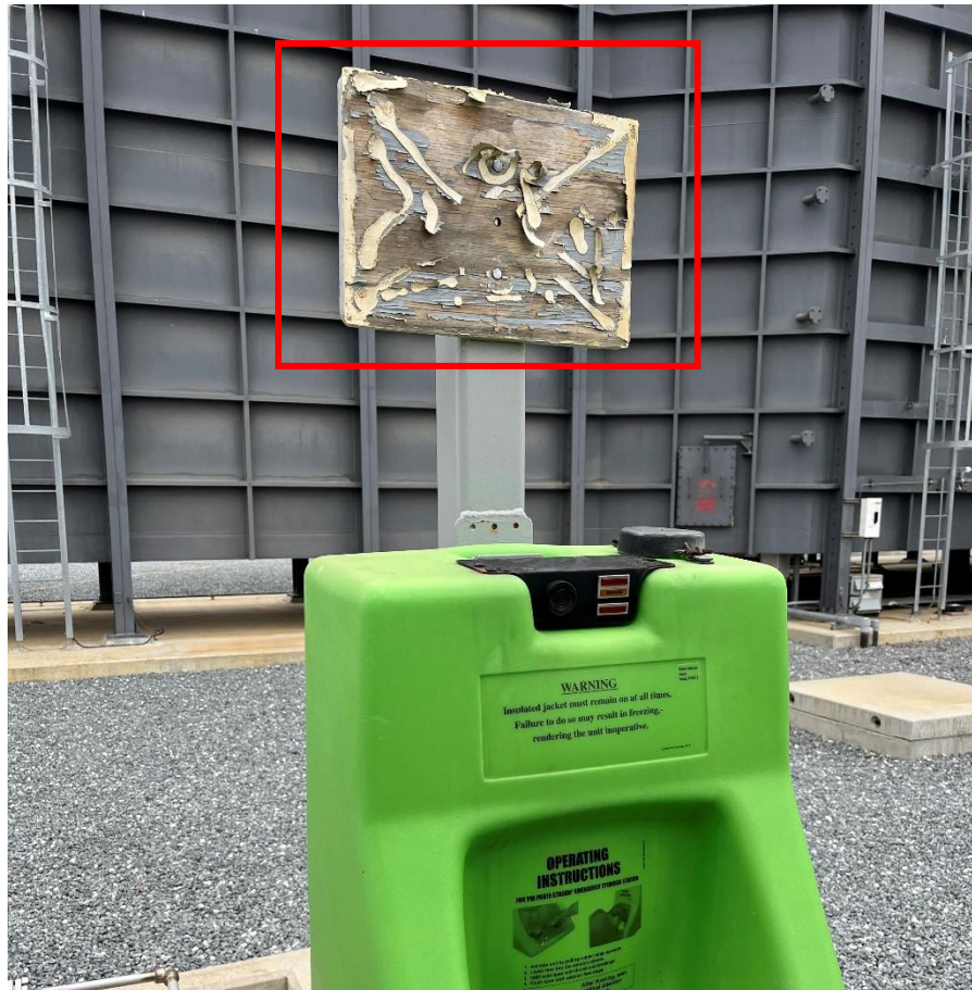
Figure 11: Damaged emergency eyewash sign
