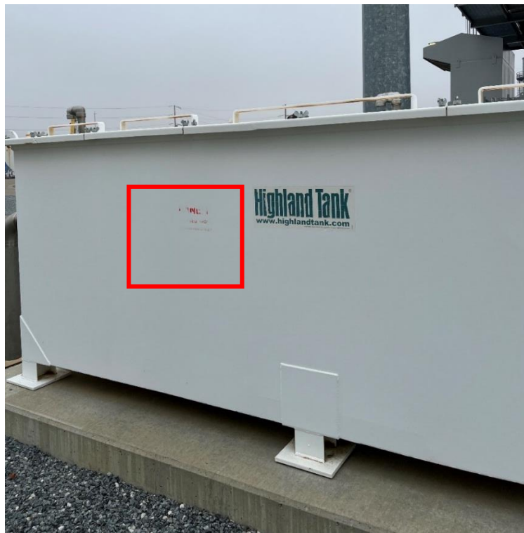
Figure 17: Oily water separator confined space label.
