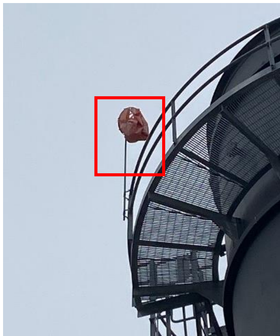
Figure 7: Deteriorated Windsock on Unit 2
