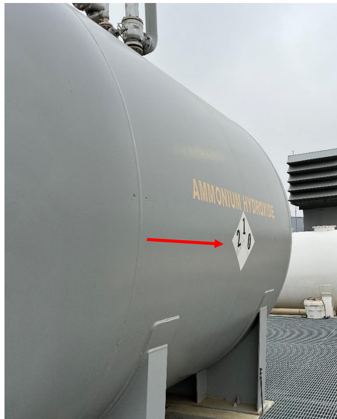
Figure 14: Ammonia Hydroxide tank
