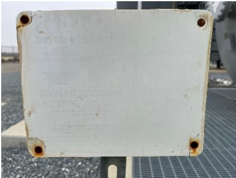
Figure 13: Faded danger sign for Ammonia Hydroxide
