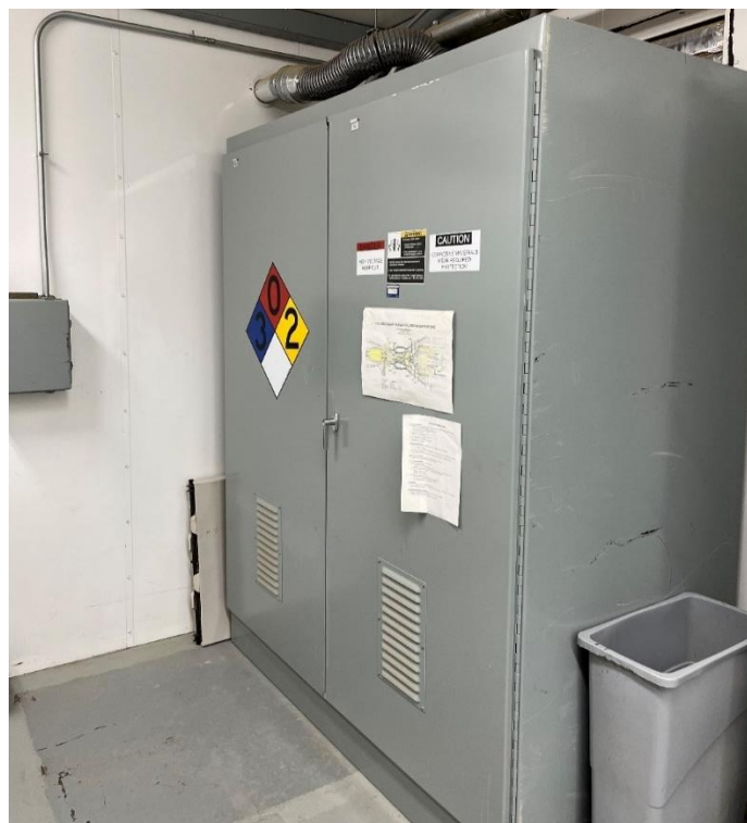
Figure 8: DC Battery Cabinet in BOP
