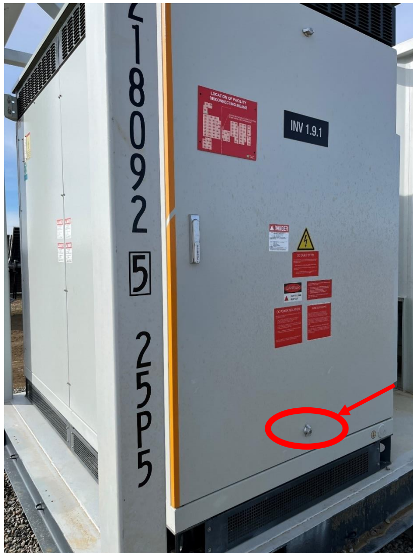
Figure 17: Inverter 1.9.1 had unlocked and unsecured cabinet
