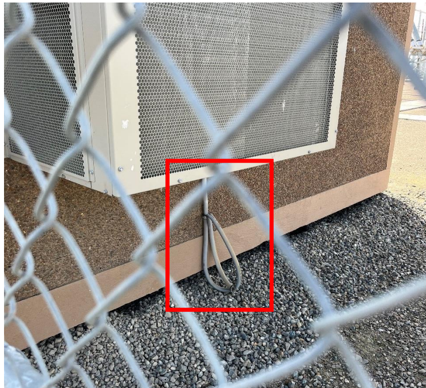
Figure 12: HVAC Drain zip tied
