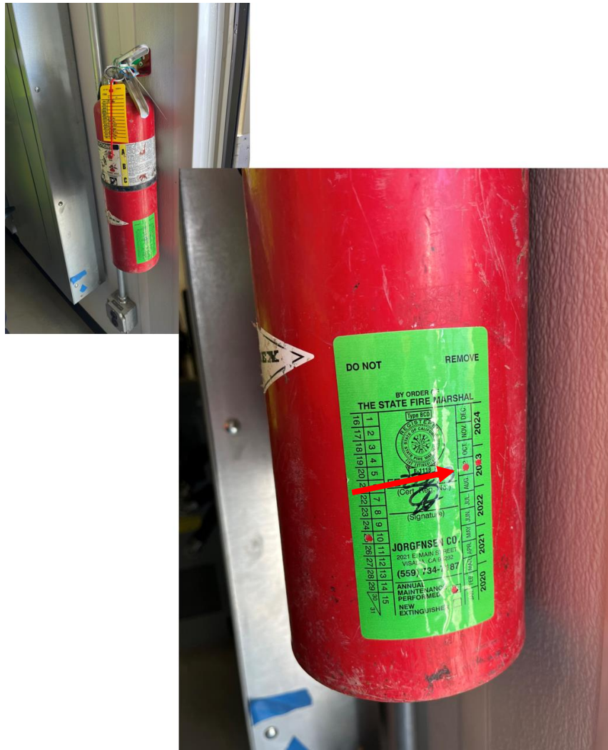
Figure 7: Fire extinguisher missing annual maintenance for 2024
