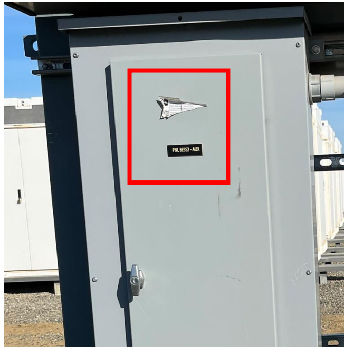
Figure 15: Warning labels on various electrical equipment throughout the site have been faded by sun.
