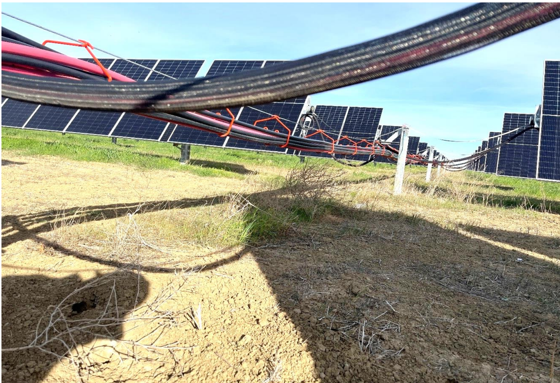
Figure 21: Vegetation Growing into Main DC Wire Run
