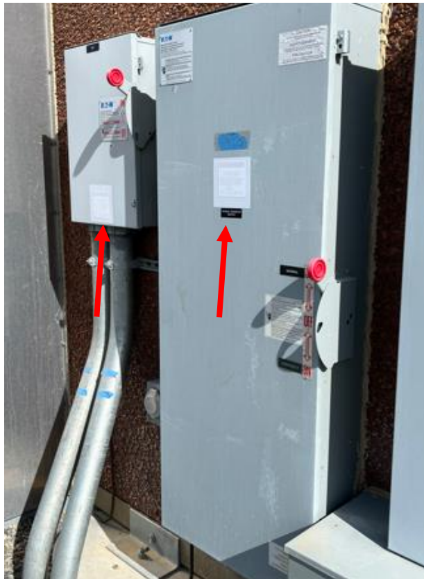
Figure 13: Warning labels faded on low voltage equipment (Substation building MTS & AC Disconnects)
