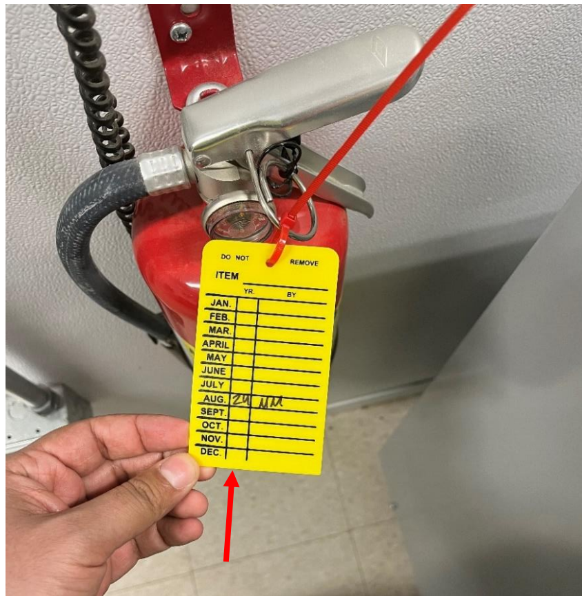
Figure 3: Fire Extinguisher missing monthly inspections
