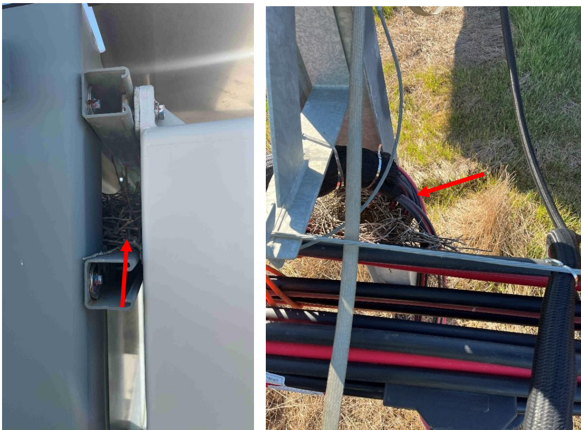
Figure 20: Nest Behind Nextracker Control Enclosure (Left) and on DC bundle (Right)
