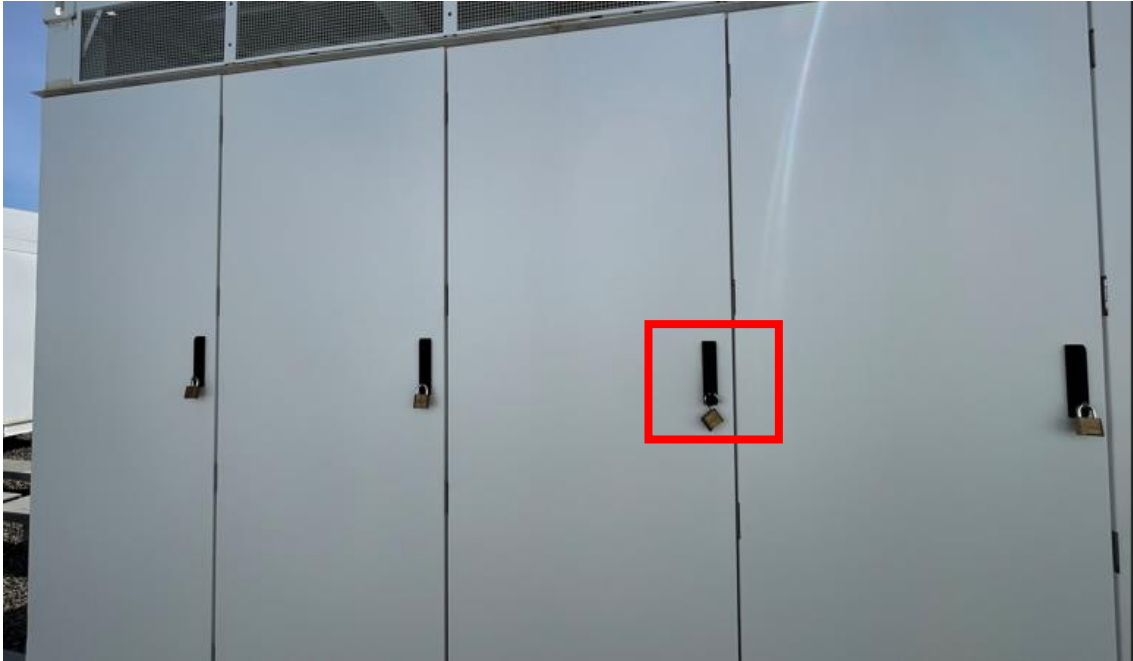
Figure 18: BESS megapack cabinets unlocked
