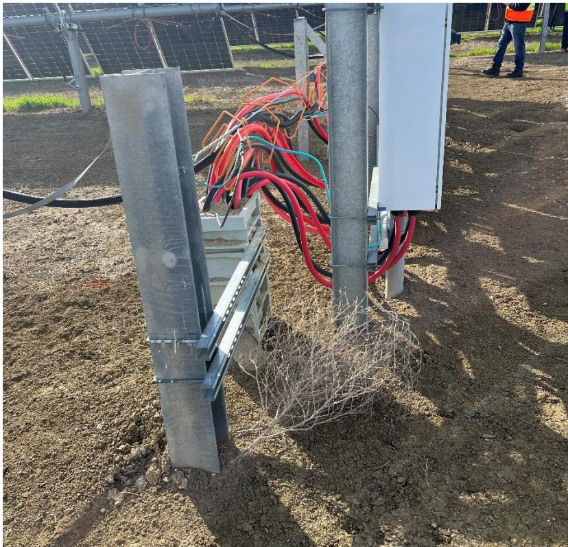
Figure 22: Tumble Weeds Adjacent to Combiner Boxes
