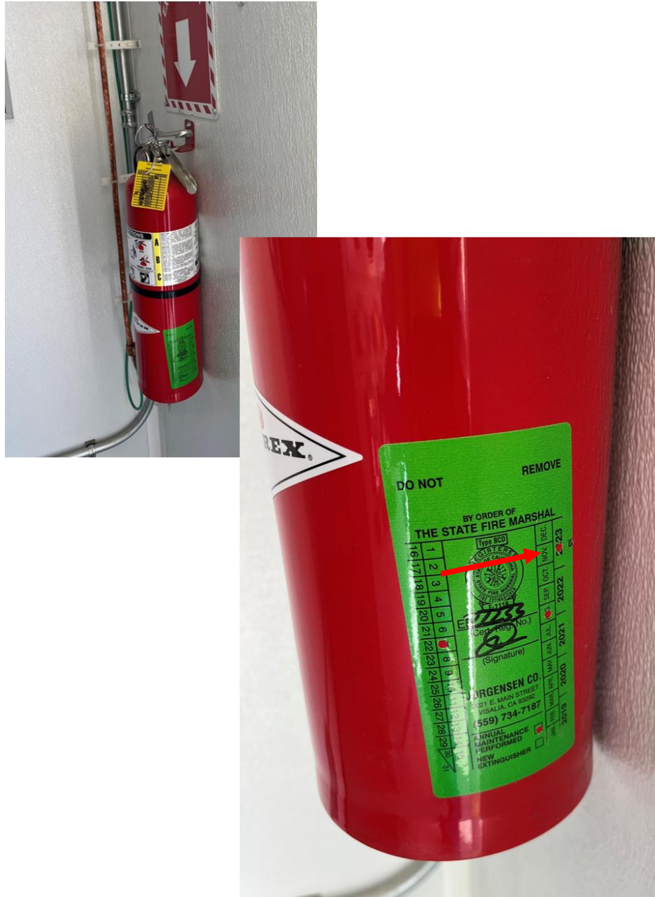
Figure 6: Fire extinguisher missing annual maintenance for 2024
