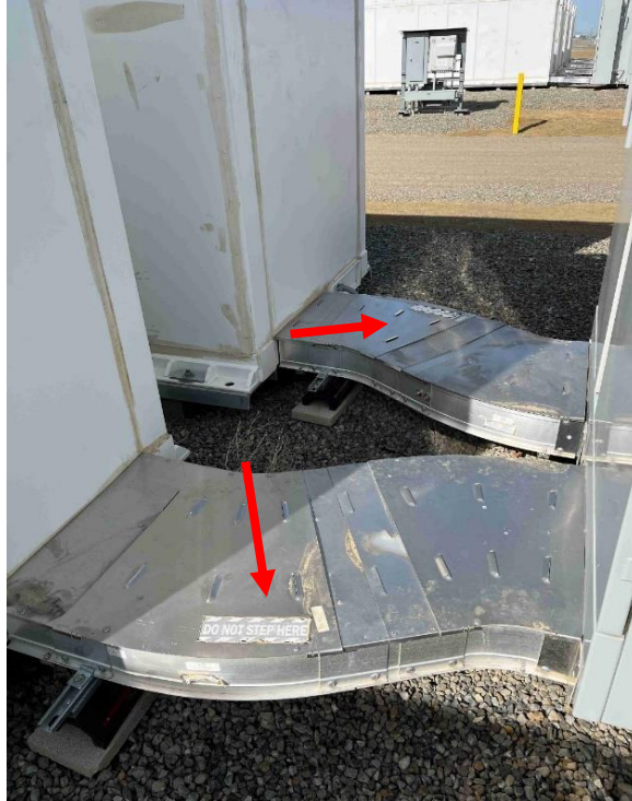
Figure 14: Tesla BESS "Do not step here" between BESS & Transformer
