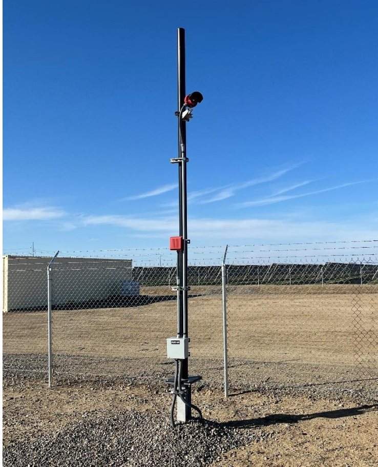
Figure 2: Example of Flame detector at Castanea BESS
