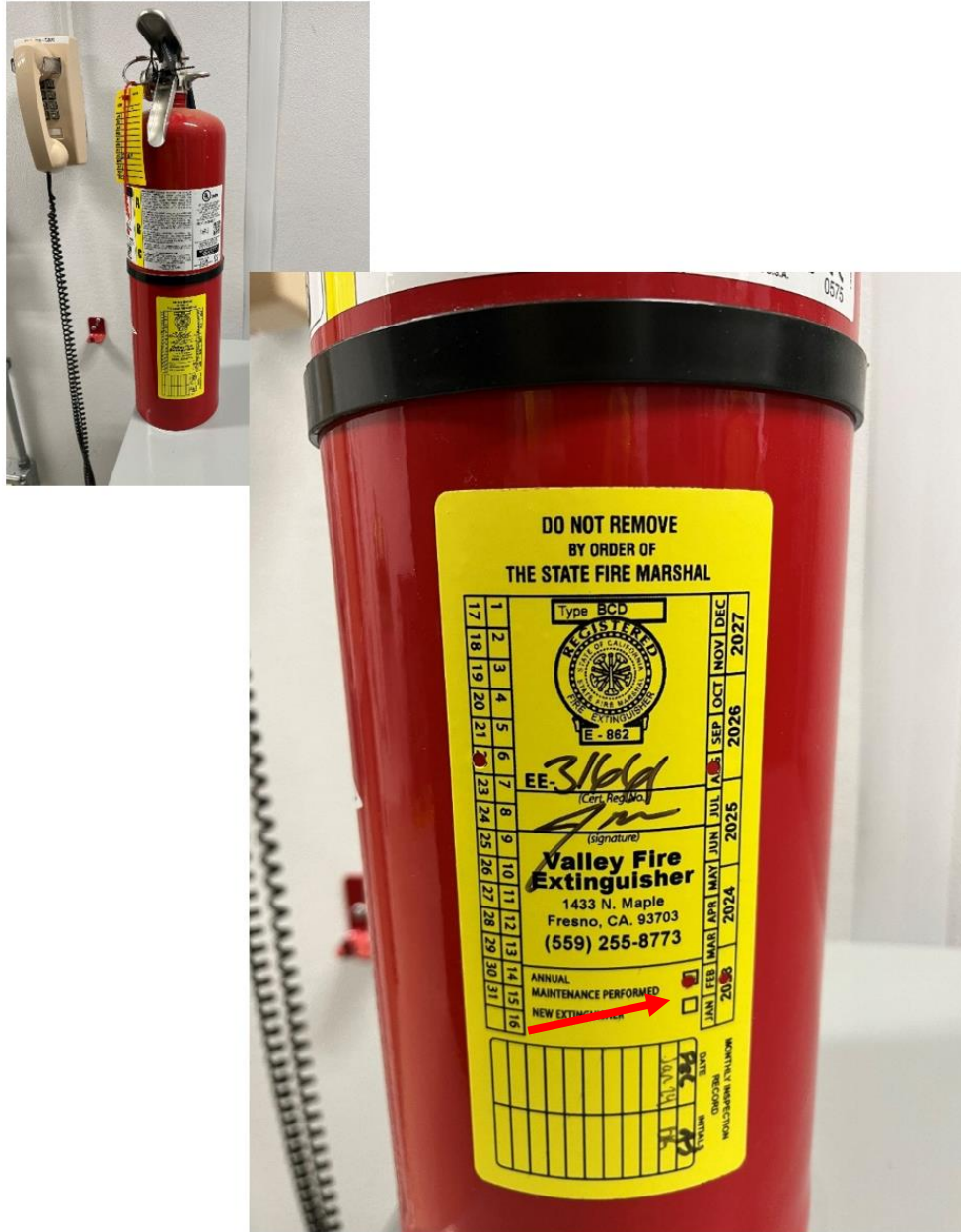
Figure 4: Fire extinguisher missing annual maintenance for 2024
