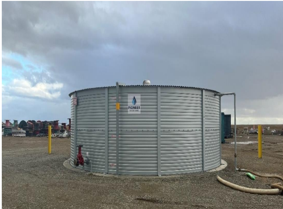
Figure 23: Water Tank without Confined Space Label
