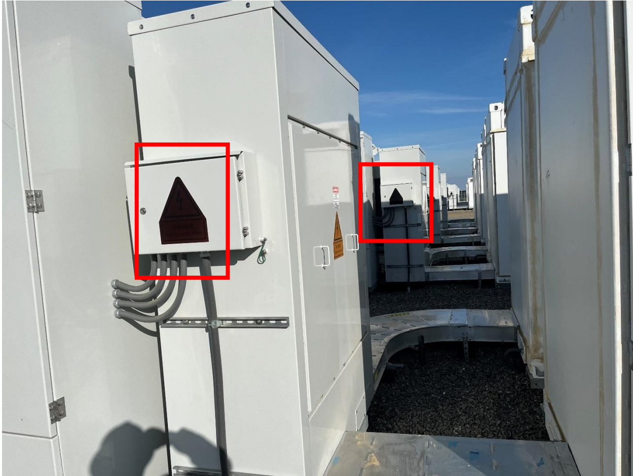
Figure 16: High Voltage Sign on BESS Transformer is illegible
