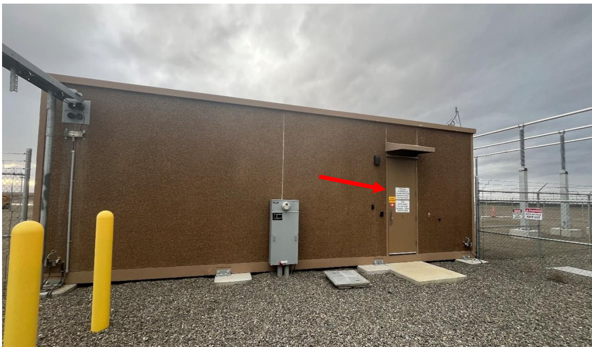
Figure 11: Castanea Project Substation Building with NFPA Placard Missing
