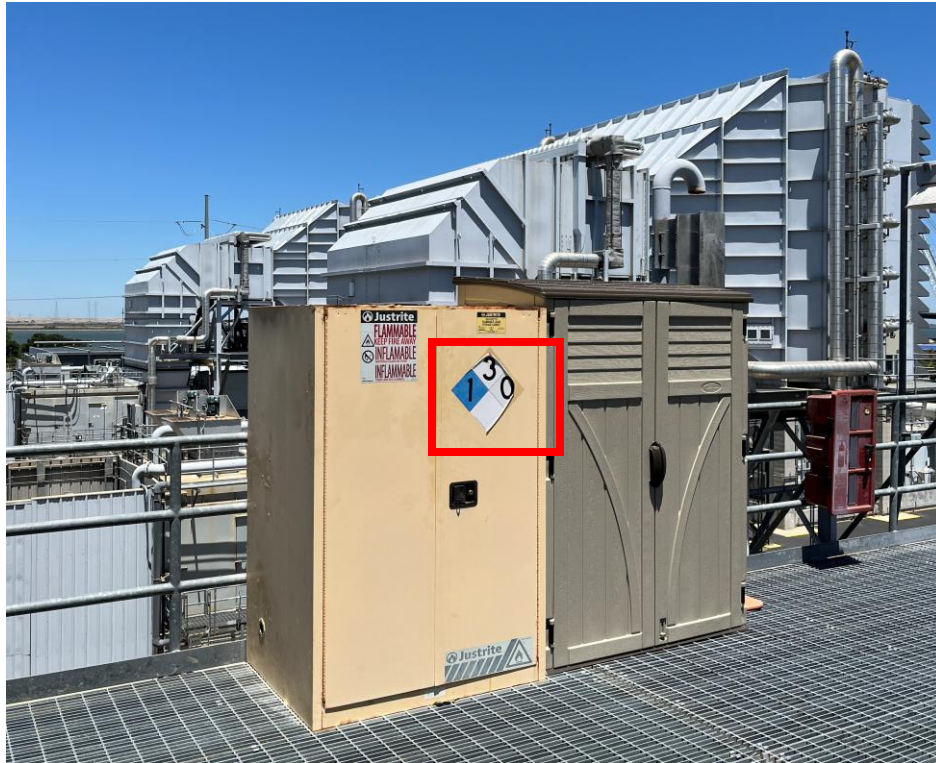
Figure 16: Color-faded on NFPA 704 Placard.
