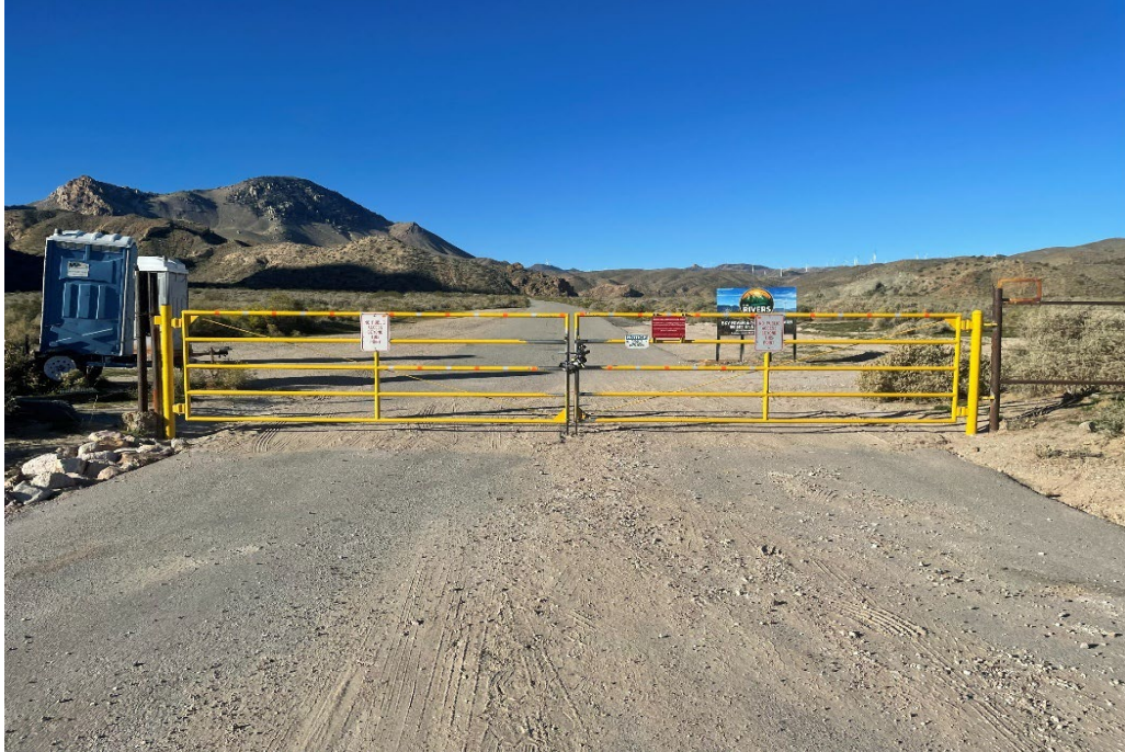
Figure 9: Main entrance gate into the site.
