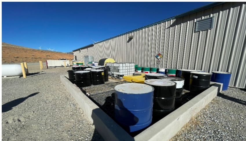
Figure 1: Hazardous waste collection area with improperly marked empty drums.
