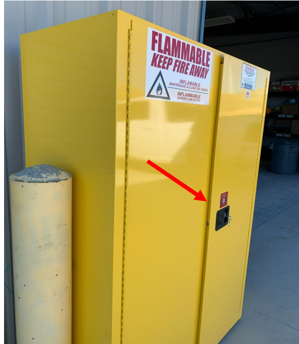
Figure 3: Flammable storage cabinet not latching.
