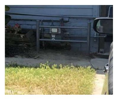
SoCalGas would disagree with SED's assessment that the meter set assembly at W. 55th, which is SoCalGas' address of record, not 55th Place, is exposed to vehicular traffic. The meter set assembly is an underset on a side of the house with no vehicular or pedestrian traffic in the area. A picture of the meter set assembly location is shown below:
