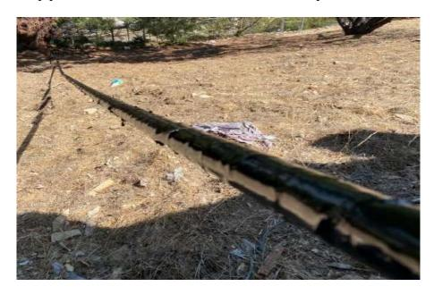
SoCalGas disagrees with SED's statement that the pipe showed signs of atmospheric corrosion. The pipe was found to have surface rust that was addressed by re-wrapping the pipe.
