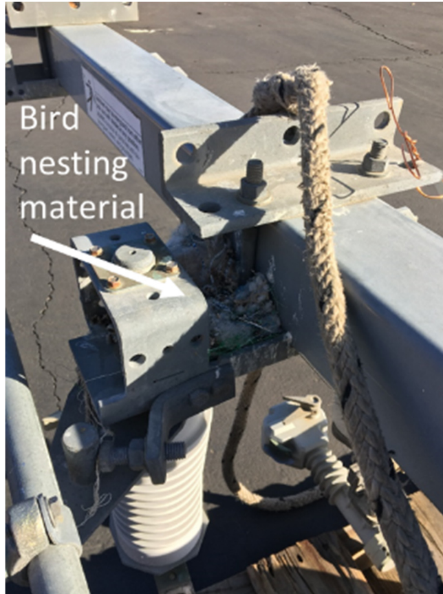
Figure 10: Bird nesting material above the section of the switch that connects the middle conductor phase of pole switch PS 2191. 56
