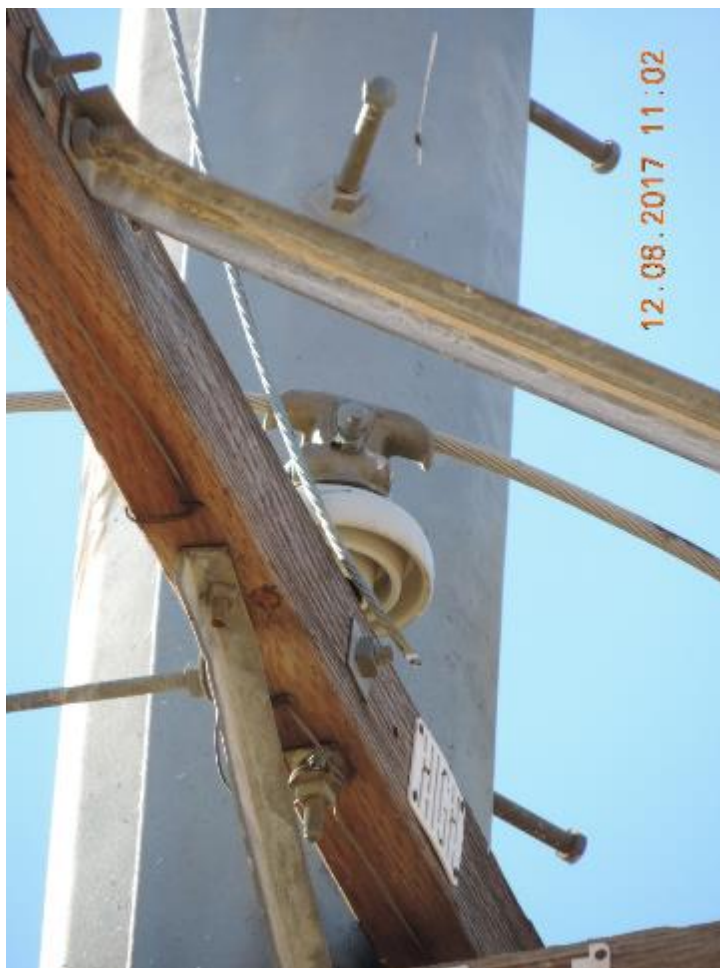
Figure 7: Free end of guy wire resting on a distribution level crossarm before evidence was removed
