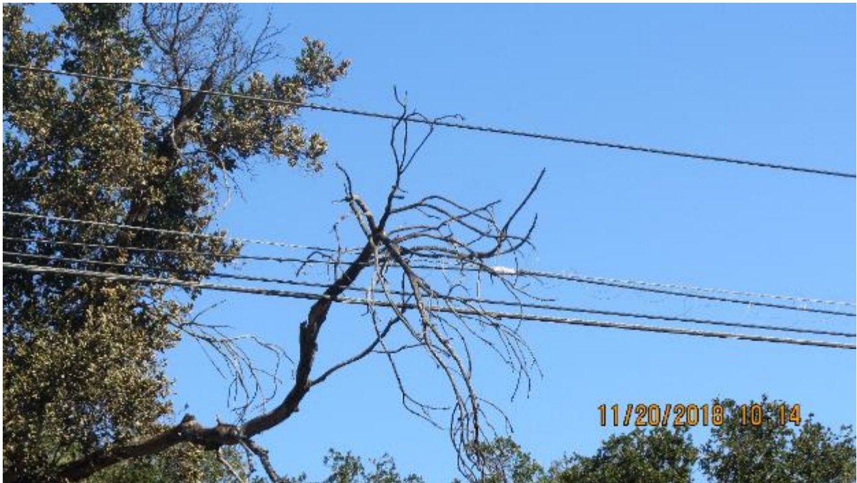
Figure 24: One of the branches pressing the communications conductors together at Site 1. 35
