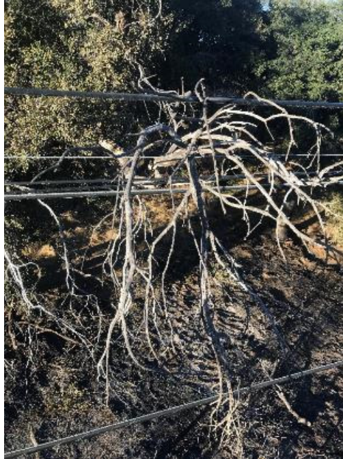
Figure 23: Another view of the overgrown tree branches pressing the communications facilities together. Viewed from an elevated position in the south. 34
