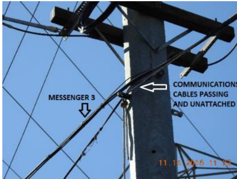
Figure 19: Communications conductors in contact with the surface of the steel pole, but not attached to it. Viewed from the northeast. 30
