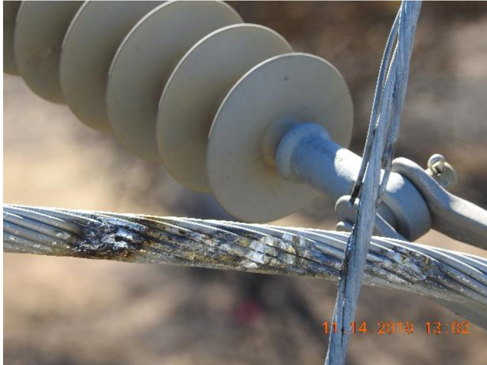
Figure 13: A detail of the damage to the jumper wire on the Steel Pole and the transmission down guy wire, Down Guy 1. 25
