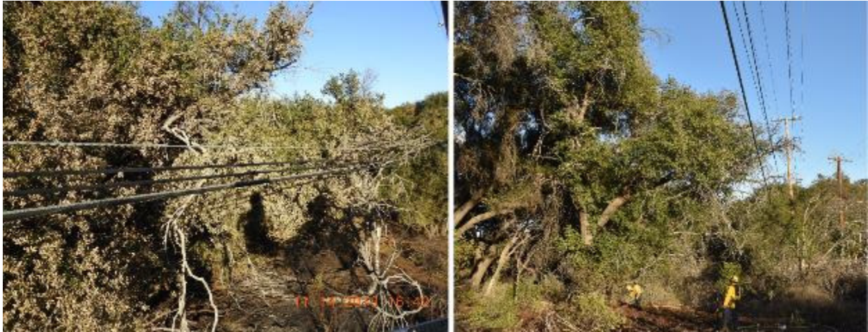
Figure 26: On the left are the communications conductors and tree branches as they appeared on November 14, 2018. On the right is a photograph taken by VCFD of the same part of the span in December 2015. 39
