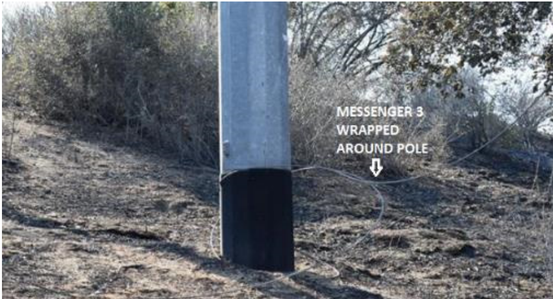
Figure 3: Messenger Wire 3 broken and wrapped around the base of the Steel Pole. 7
