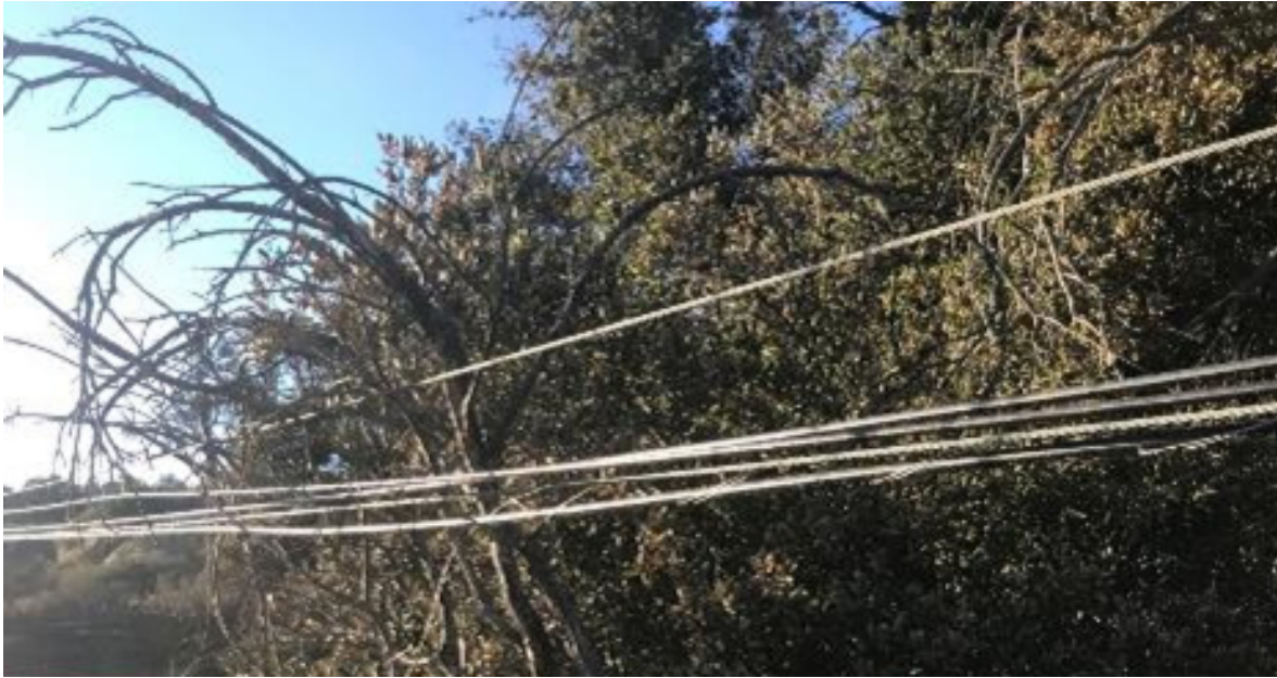
Figure 7: Overgrown tree branches pressing the ECS communications conductor into the third-party communications conductor at Site 1. The communications conductors separated from their messenger guys when their lashing wires melted during the arcing event. 14
