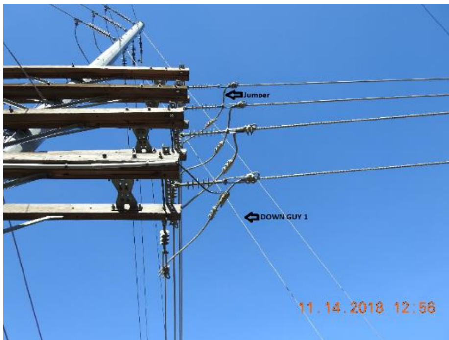
Figure 14: The jumper and down guy that made contact as viewed from the base of the Steel Pole. 26
