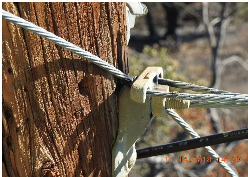
Figure 18: A detail of the distribution down guy, Down Guy 2, in contact with Messenger Wire 1 and the through bolt on the Stubbed Pole. Note the blackened area on the down guy and the Stubbed Pole at the point of contact. 29
