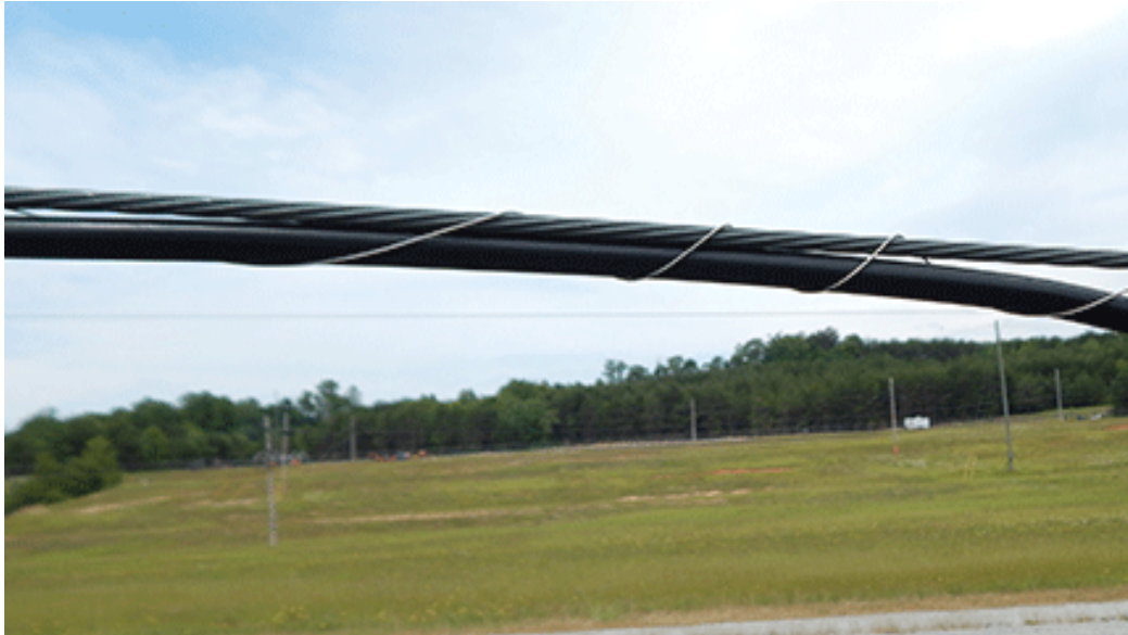
Figure 4: A messenger wire supporting a communications conductor and wrapped with lashing wire. Note that this is a stock image and that this particular communications conductor was not involved in the Woolsey Fire in any way. However, the communications infrastructure involved in the Woolsey Fire was very similar to that depicted in the image.
