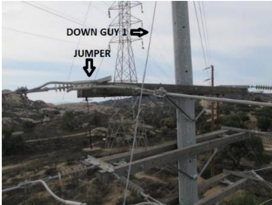
Figure 11: A lateral view of Down Guy 1 and the jumper wire taken from an elevated work platform from the northeast. 23
