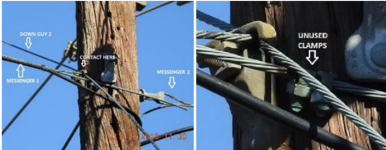
Figure 6: The top of the Stubbed Pole as viewed from the southwest. Note the unattached bonding extension on Messenger Wire 1 in the photograph on the left. On the right is a detail of the extension showing the unused bonding clamps. 9
