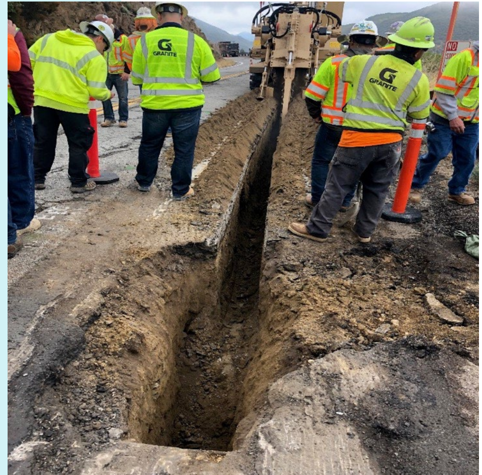
Tesmec Trencher civil construction – Sunrise Highway, Mount Laguna
