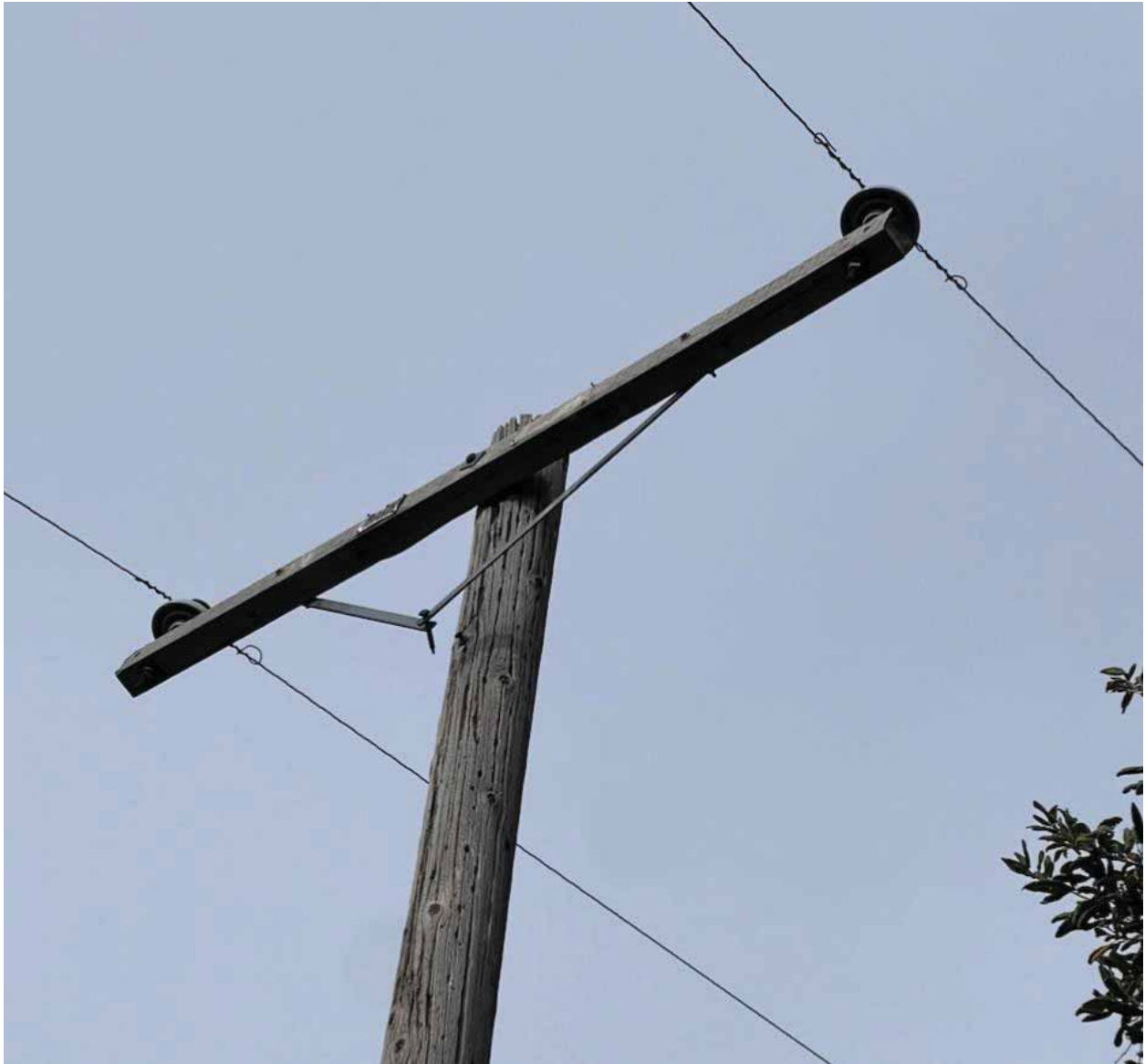
Figure 26 - Item #9 P166012 Crossarm Brace and Bolt Damage
