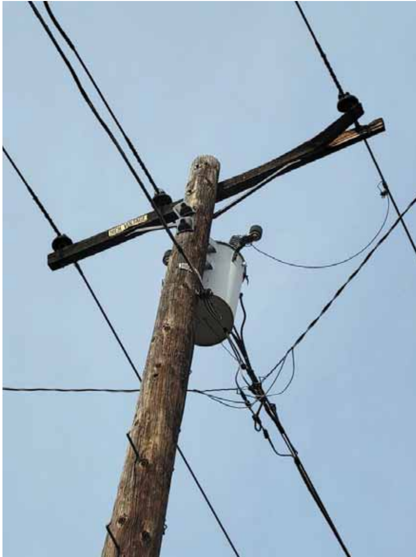
Figure 23 - Item #6 P516439 Damaged Crossarm
