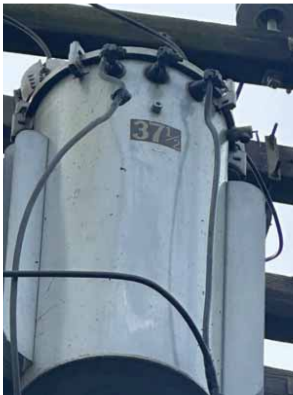
Figure 20 - Item #3 P213996 Leaking Transformer
