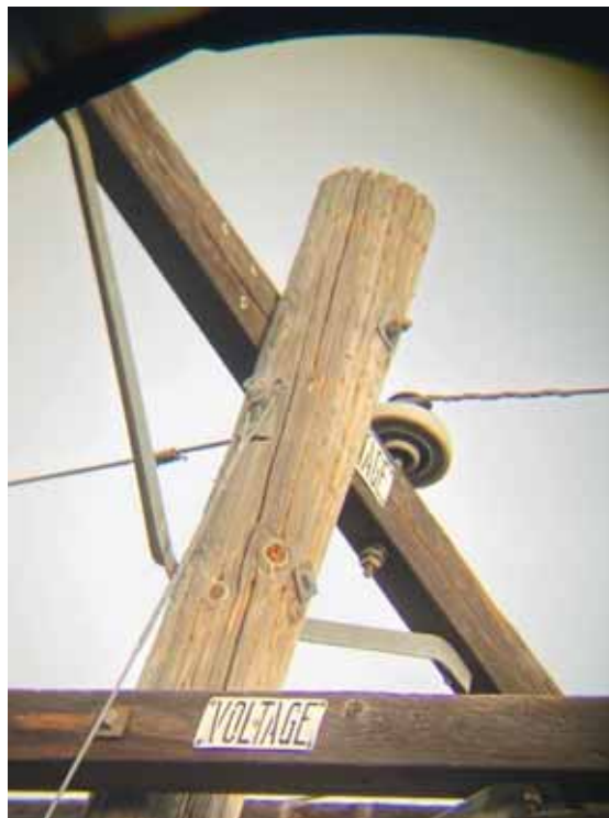
Figure 21 - Item #4 P119515 Damaged Crossarm
