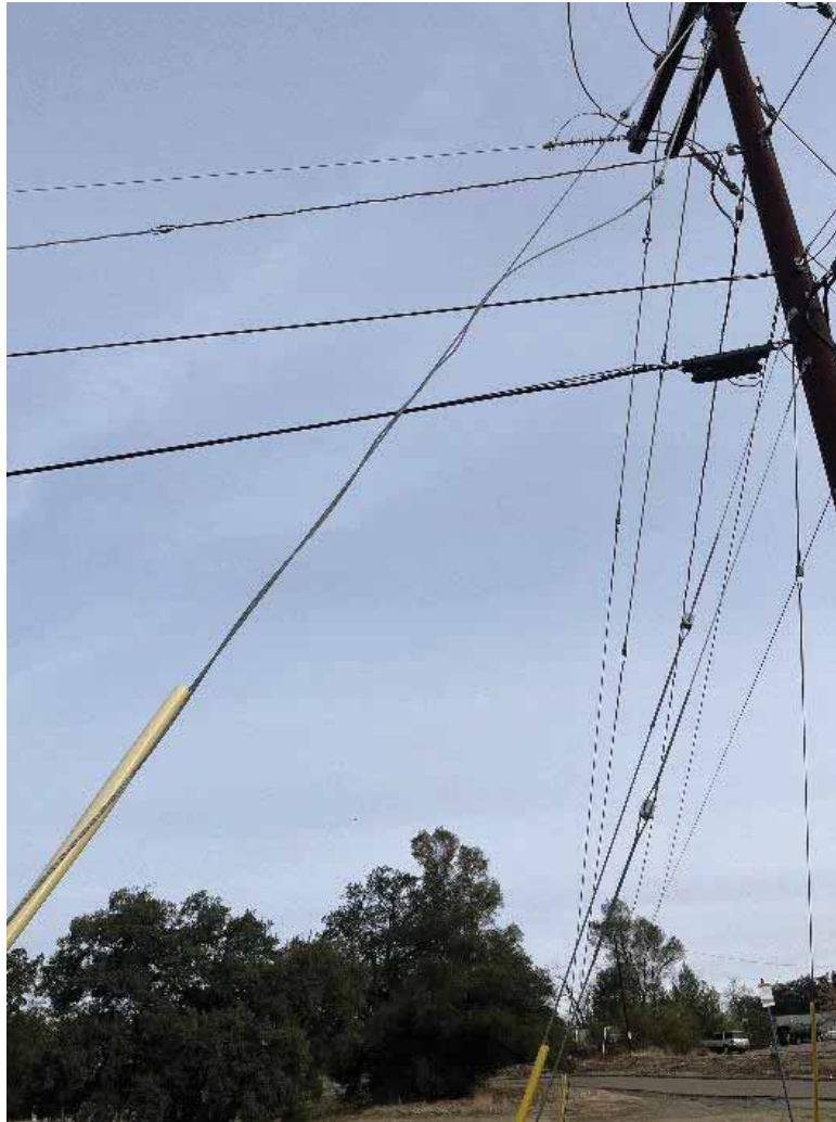
Figure 24 - Item #7 P78896 Broken Down Guy
