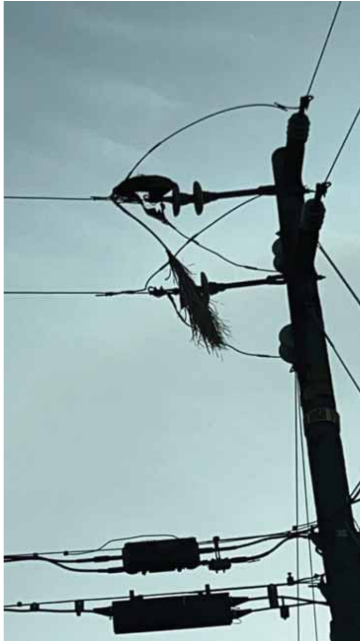
Figure 22 - Item #5 P419391 Palm Frond Landed on Primary Wire
