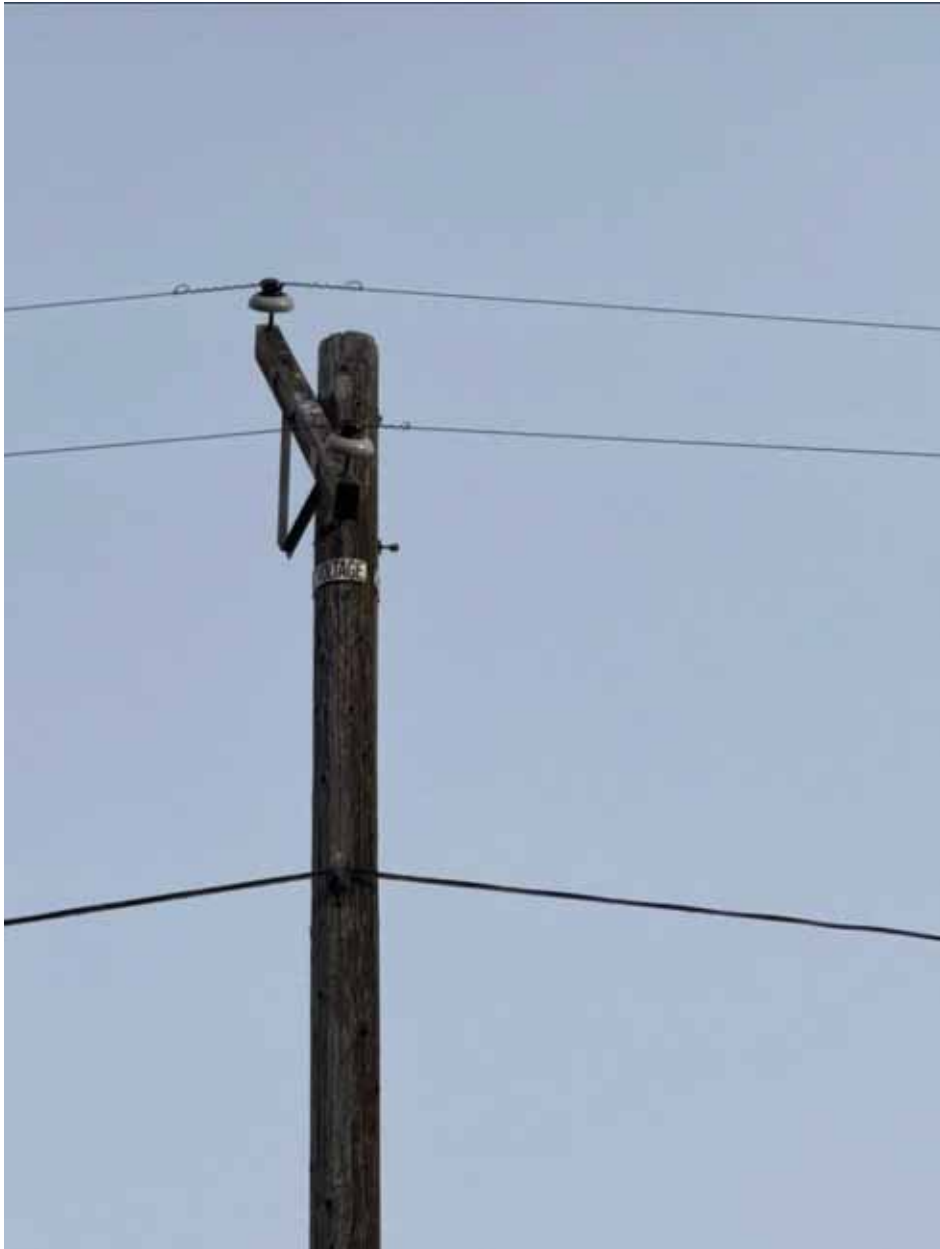
Figure 19 - Item #2 P376436 Crossarm Brace and Bolt Damage
