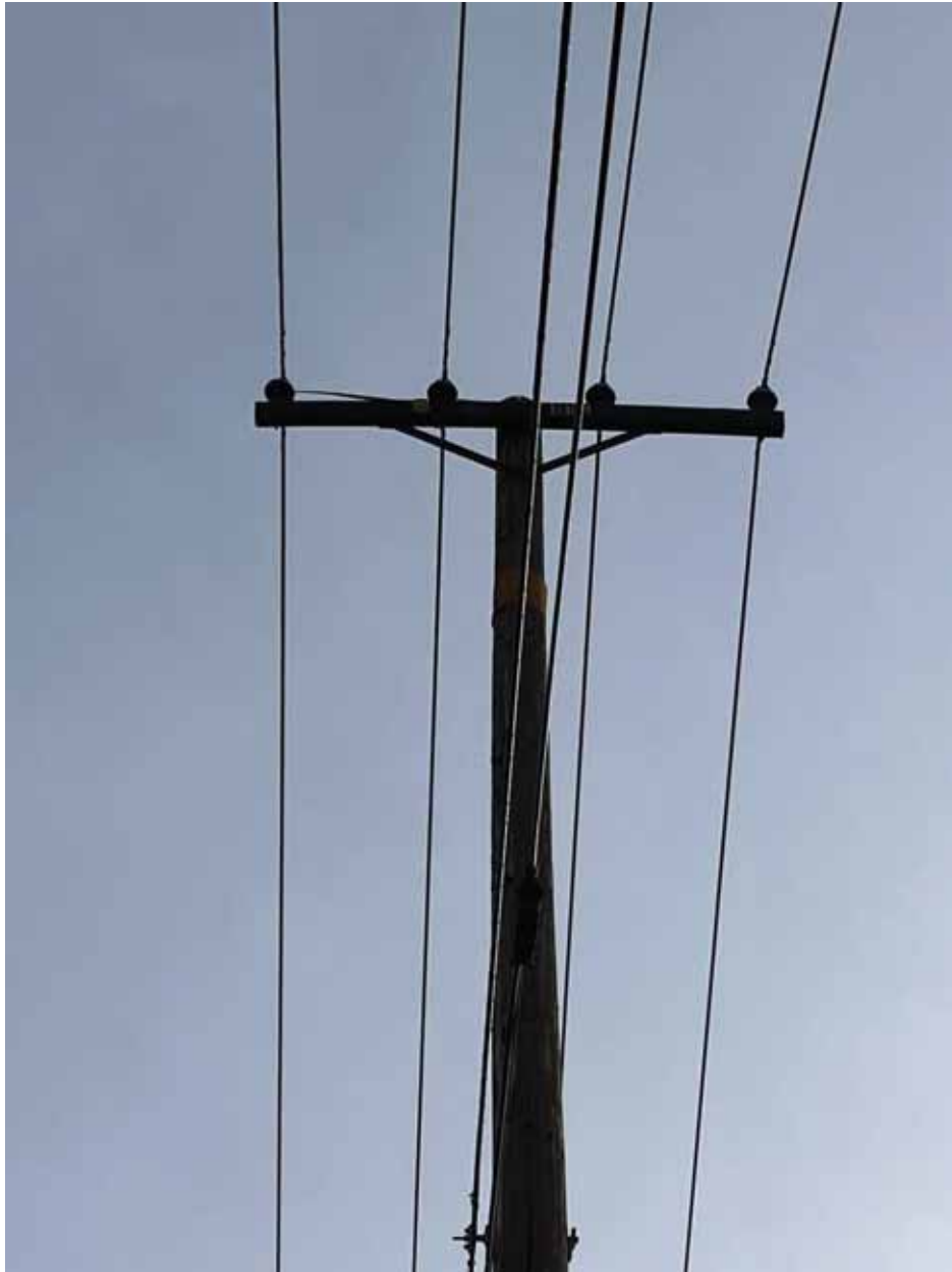
Figure 25 - Item #8 P78880 Damaged Crossarm
