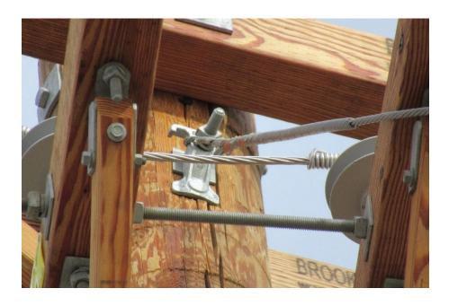
Figure 1: Down guy in proximity to the neutral conductor
