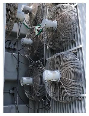
Clayton04: Abandoned cooling water hose at the transformer bank cooling fans
