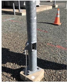
WillowPass01: At 21 kV yard - missing cover on light pole foundation
