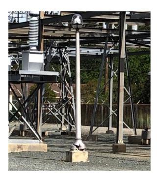
Clayton03: Damaged light pole foundation
