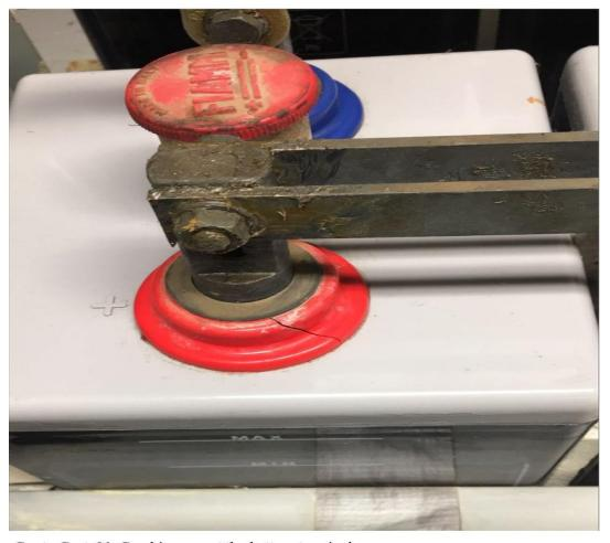
ContraCosta01: Cracking cap at the battery terminals
