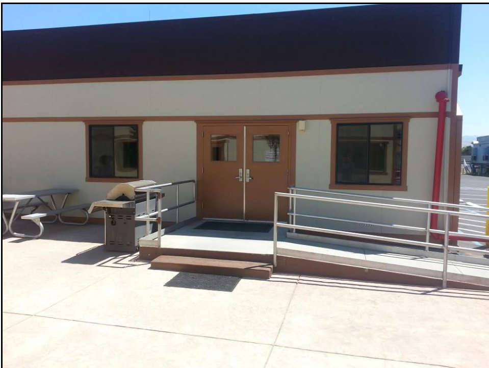
Photo 4: Reconfigured ramp to mitigate trip hazards.
