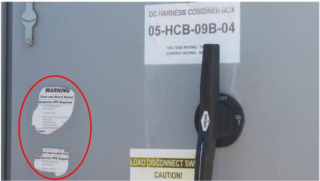
Figure 4: Partially-peeled and faded arc flash warning labels on a combiner box.
