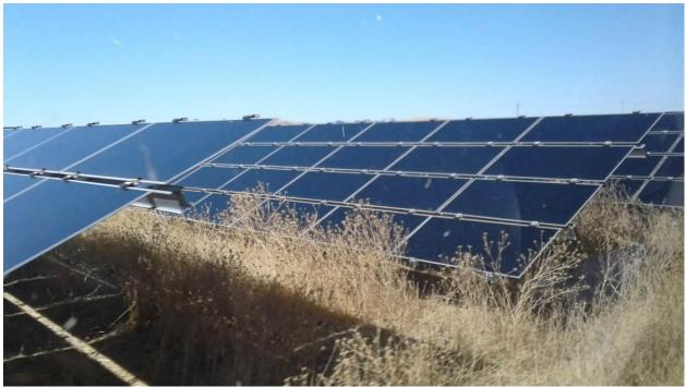
Figure 2: ESRB observed overgrown vegetation of at least several feet tall, some of which encroaches onto the solar panels.
