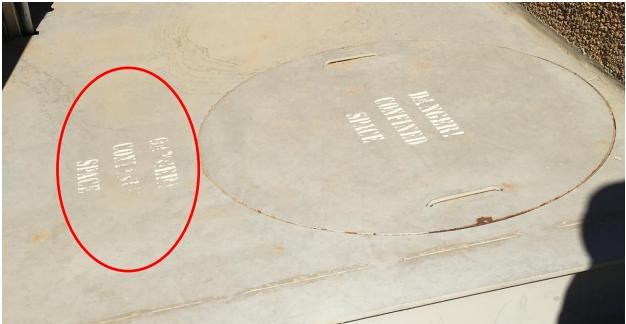
Figure 5: Faded confined space label adjacent a medium voltage transformer.
