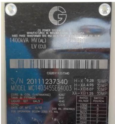
Figure 13: The nameplate on the medium voltage transformer shows it uses 627 gallons of insulating oil.
