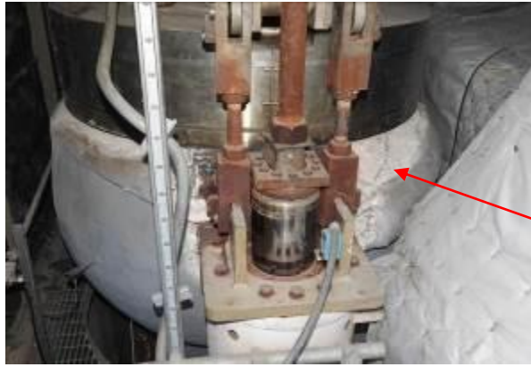
Damaged insulation and cowlings in the IP Steam Turbine Combined Reheat and Intercept Valve
