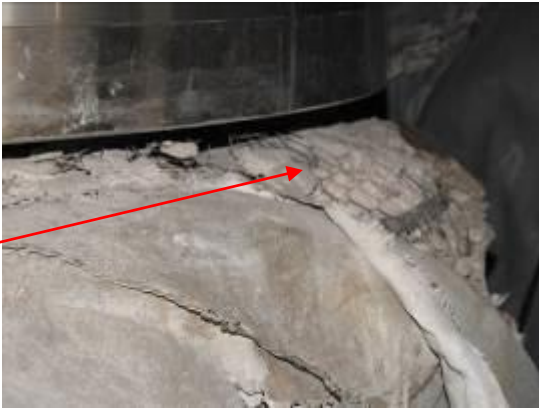
Damaged insulation and cowlings in the IP Steam Turbine Combined Reheat and Intercept Valve
