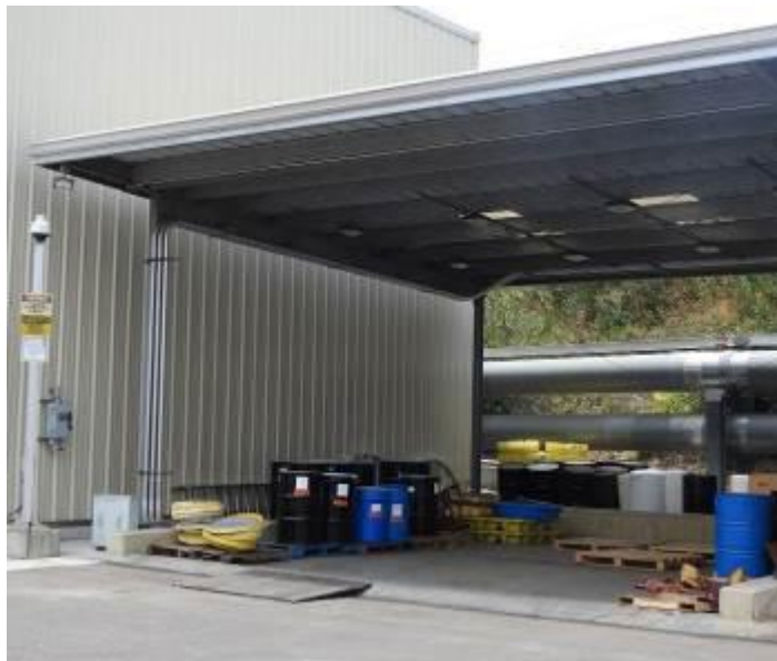
No NFPA signage on the hazardous material storage shed
