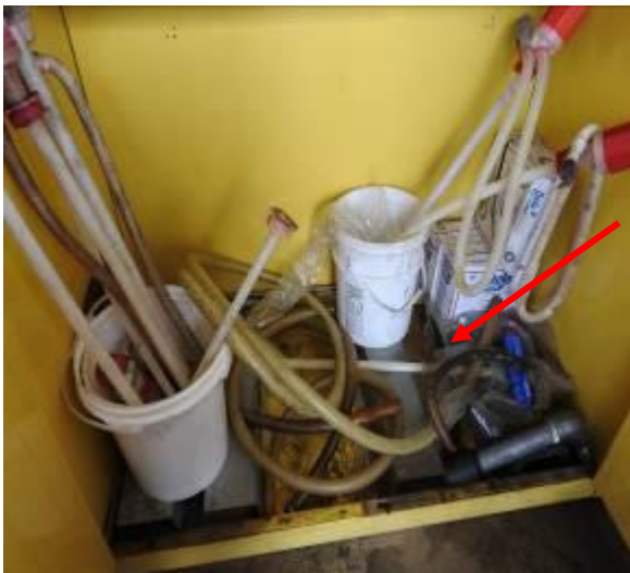
Loose pipes, empty buckets kept inside the chemical cabinet
