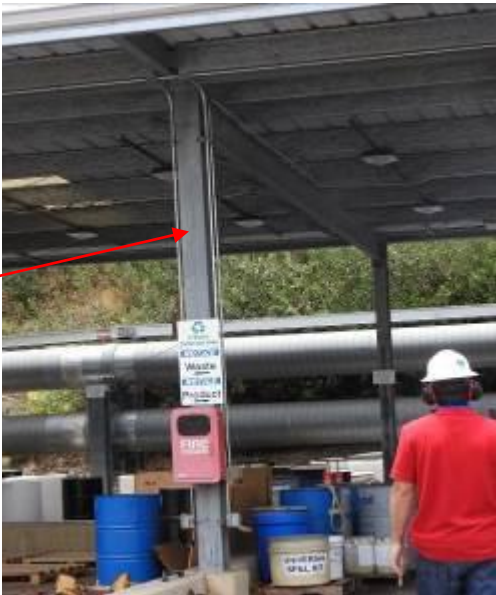
No NFPA signage on the hazardous material storage shed
