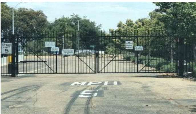
Missing NFPA Placard on the main gate.
