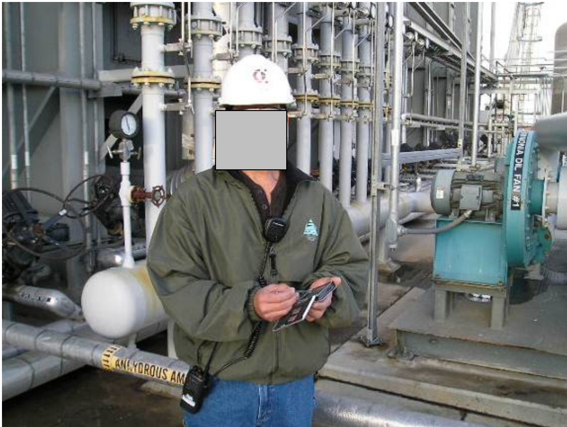
Photo 32: A roving operator seen with the digital personal assistant used for gathering plant information during routine walk downs.
