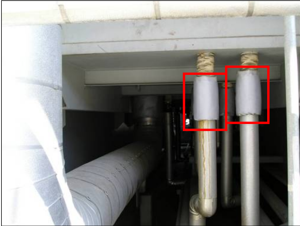
Photo 7: The plant added new piping insulation throughout the HRSG where it previously detected excessive heat leakage.
