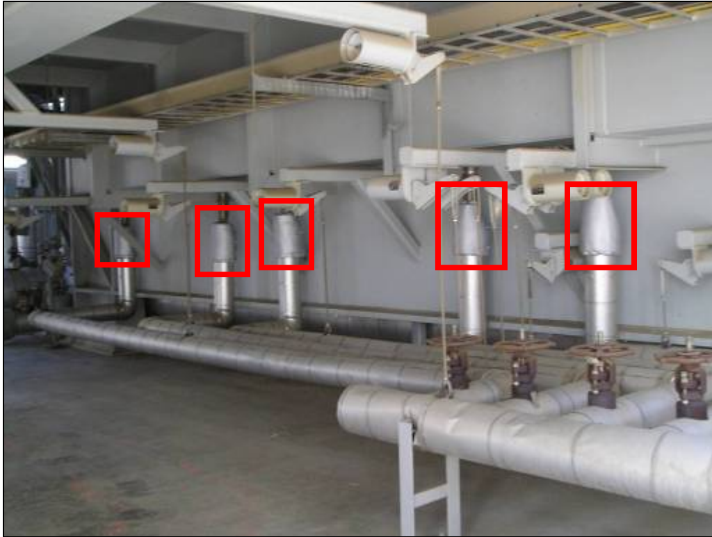
Photo 8: The plant added new piping insulation throughout the HRSG where it previously detected excessive heat leakage.
