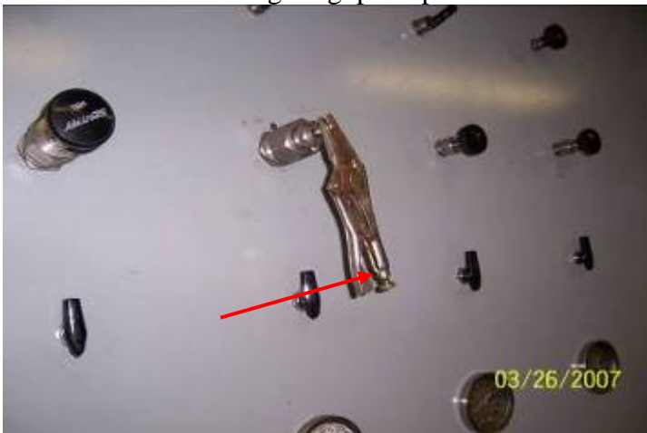
Photo 16: A vise grip is used as handle to operate the sample valve.
