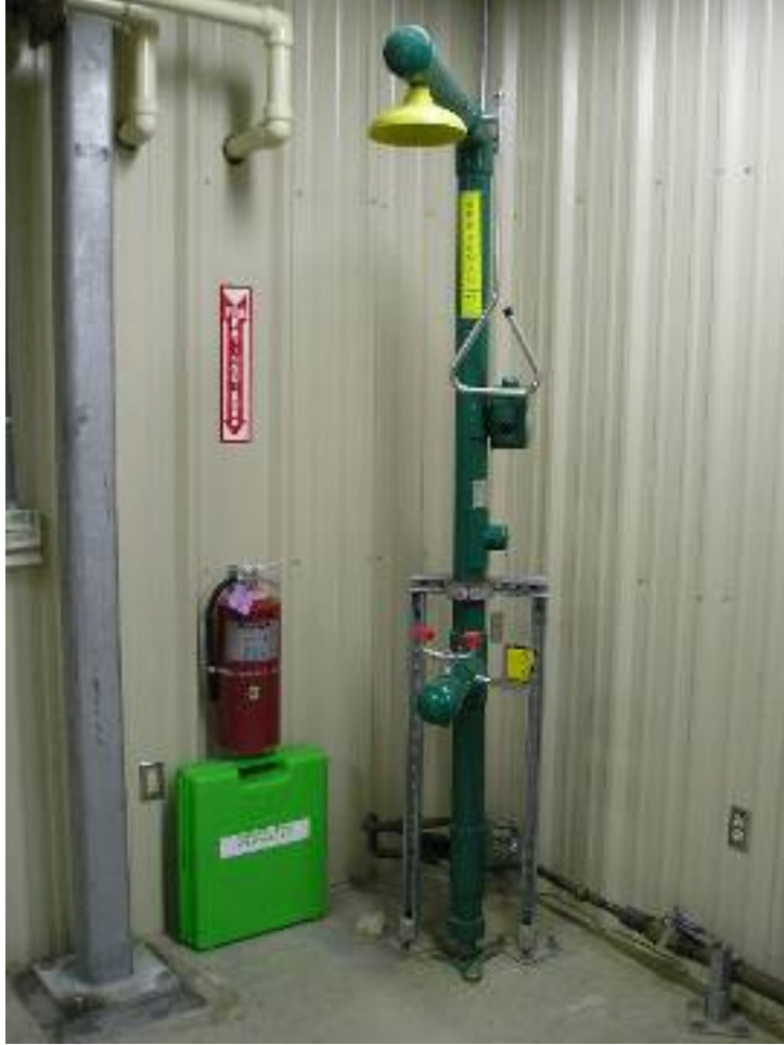
Photo 26: Emergency shower and personal protective equipment and spill containment materials are readily available.
