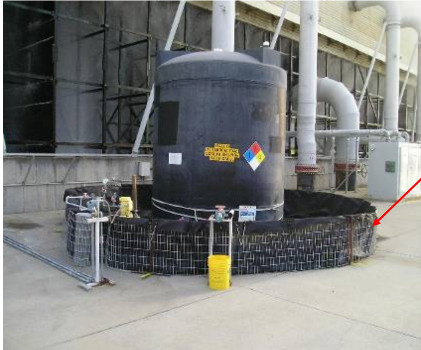
Photo 19: Temporary sodium bromide chemical injection system.
