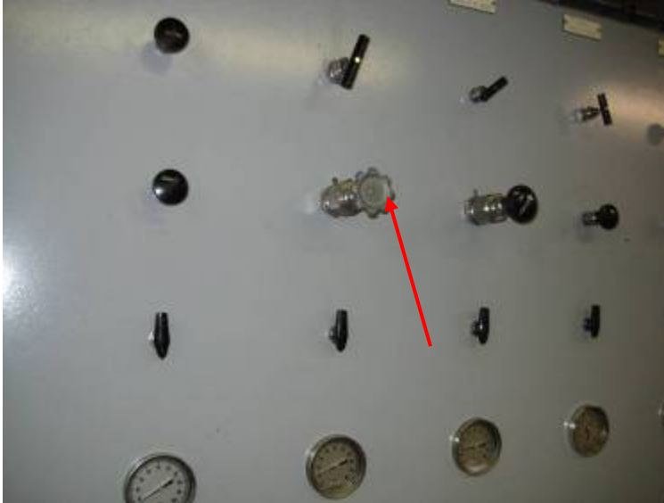
Photo 17: A new valve handle has been installed.
