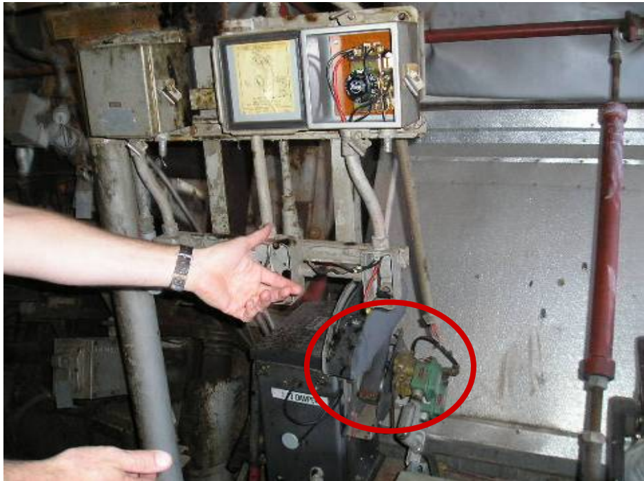
Photo 1 Uncovered wiring
