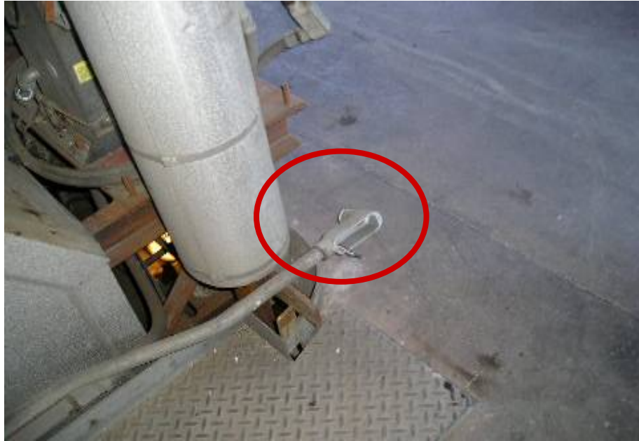
Photo 2 Uncovered wiring
