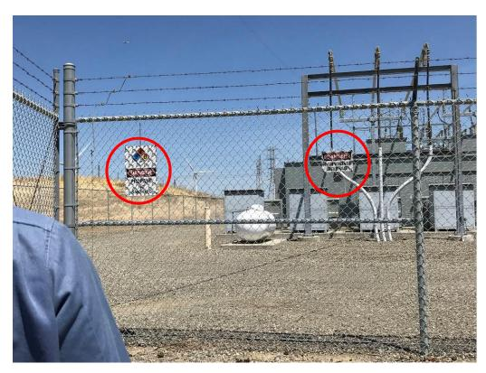
Figure 6: Warning placards visibly obstructed by chain link fence.
