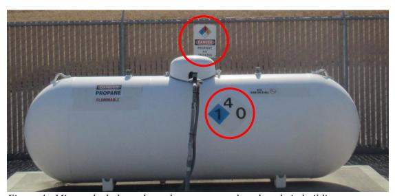
Figure 4: Mismatched placards on the propane tank at the admin building.
