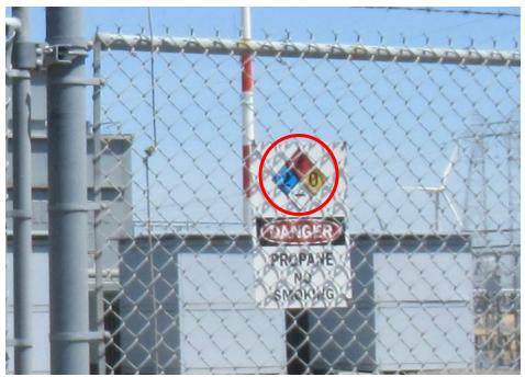
Figure 5: Mismatched placards at the substation.
