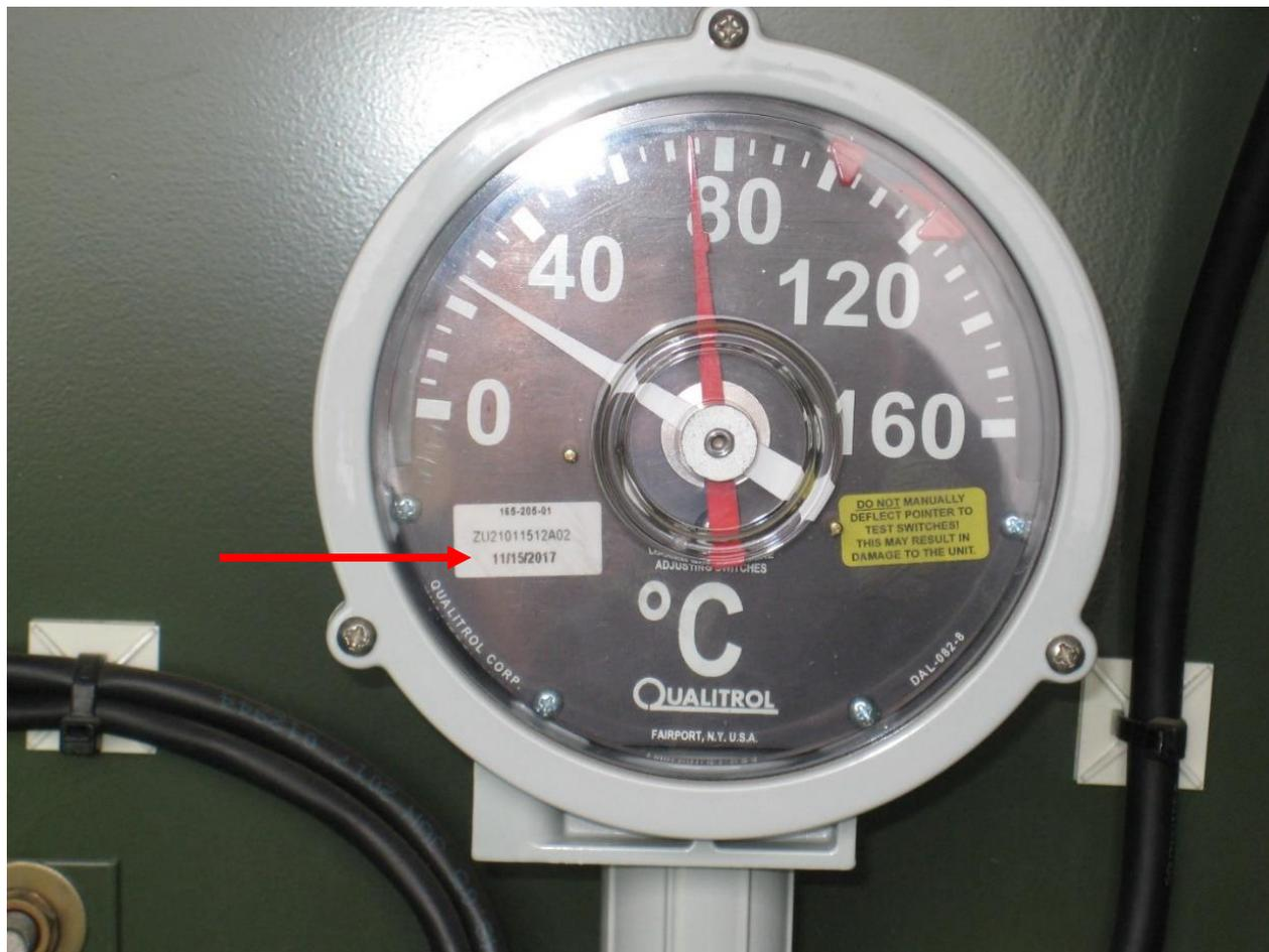
Figure 2: Transformer Temperature Gauge with a calibration sticker dated November 15, 2017. Critical gauges should be calibrated annually.
