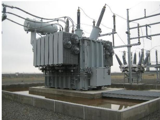
Figure 20: Existing Sept-up Tansformers w/o Sprinklers
