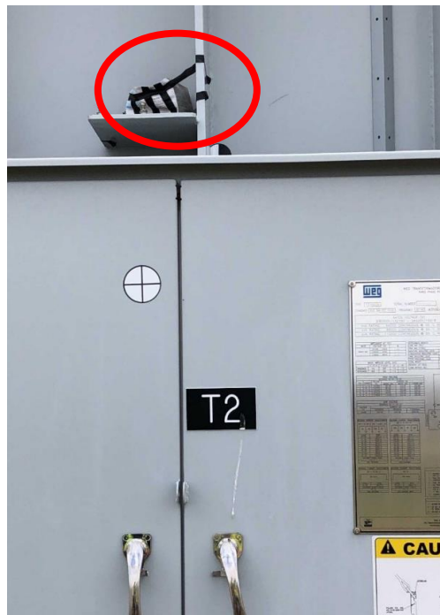
Figure 17. An unidentified foreign object taped to GSU 2.
