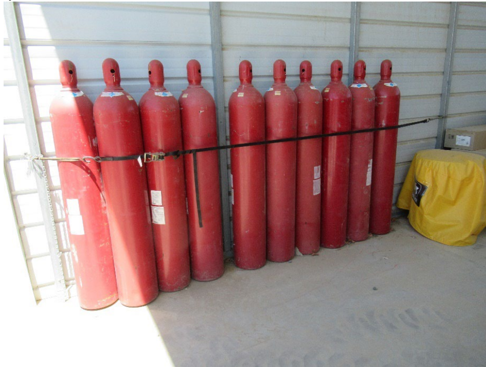
Figure 4 : Cylinders in the storage area are not equipped with two forms of securement.
