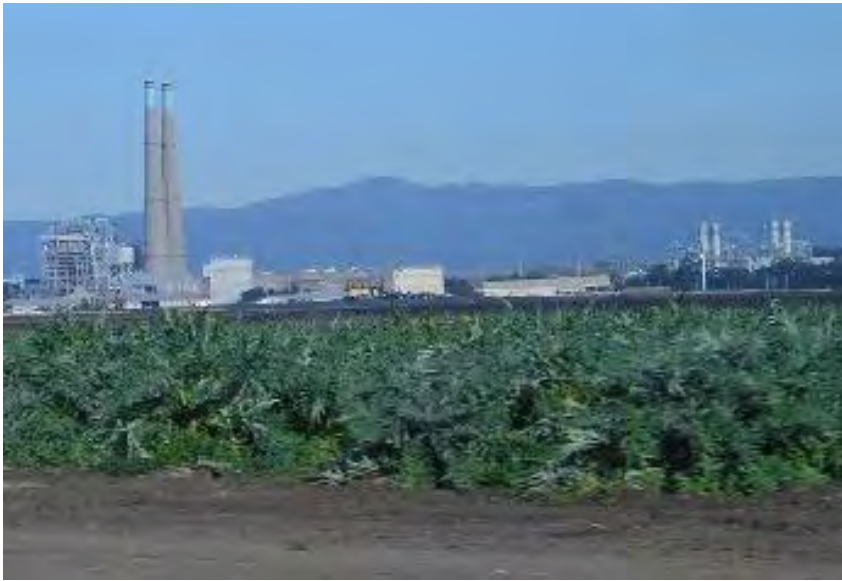
Figure 1 -- Moss Landing Power Plant as seen from Highway 1.
