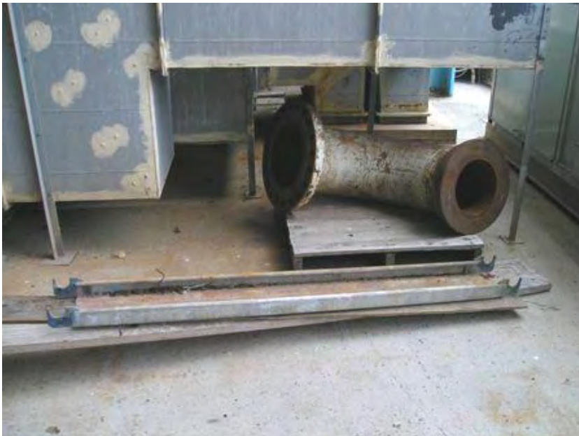
Figure 5 -- Disused piping and scaffolds accumulating on Level 104 of Units 6 and 7.
