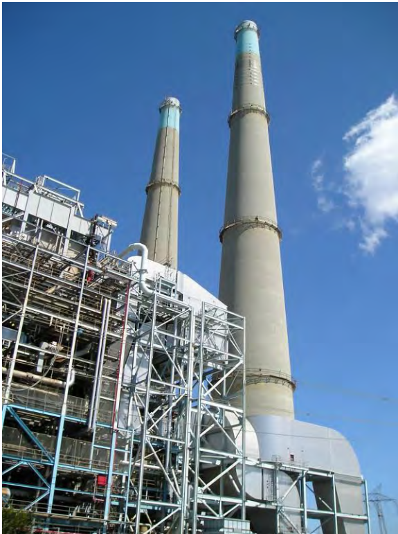
Figure 3 -- Units 6 and 7; conventional, once-through, supercritical boiler units.
