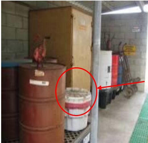
Photo 31: Spill kit in the Drum Lube Oil Storage area
