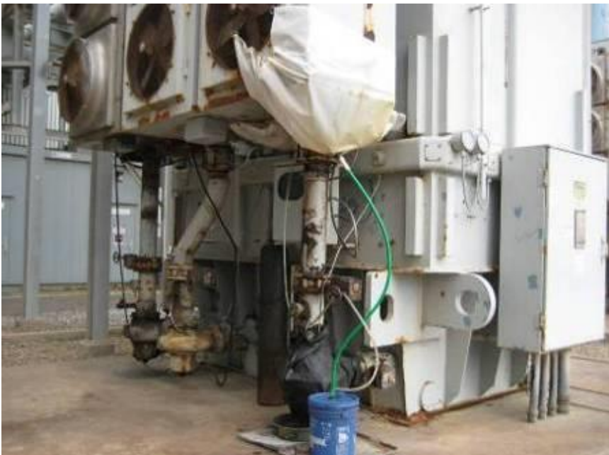
Photo 5: Completed containment mitigations, Unit 2 Phase C transformer.
