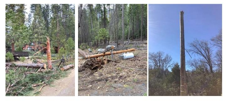
Figure 17: Wind-Caused Damage in Mariposa County - Pole Brought Down at Base, Line Down
