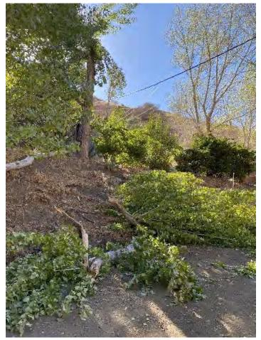
Figure 20: Vegetation-Damage in Kern County – Tree fell on Service Line
