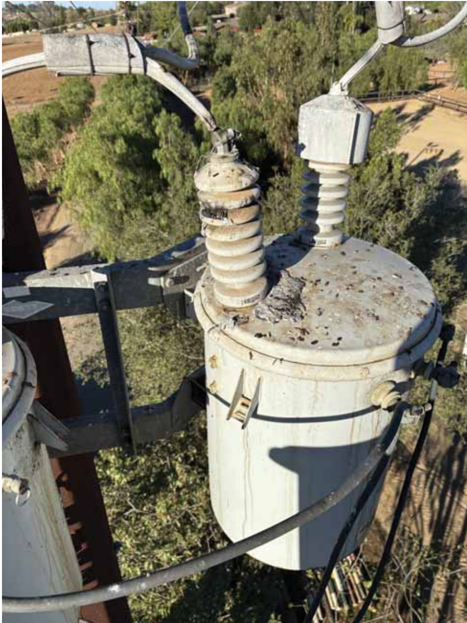
Figure 36 - Item #5 Z514166 Transformer Damage
