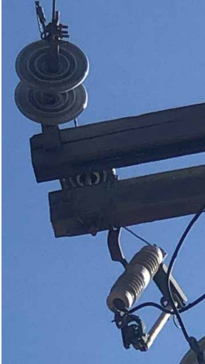
Figure 34 - Item #3 P228317 Damaged Crossarm
