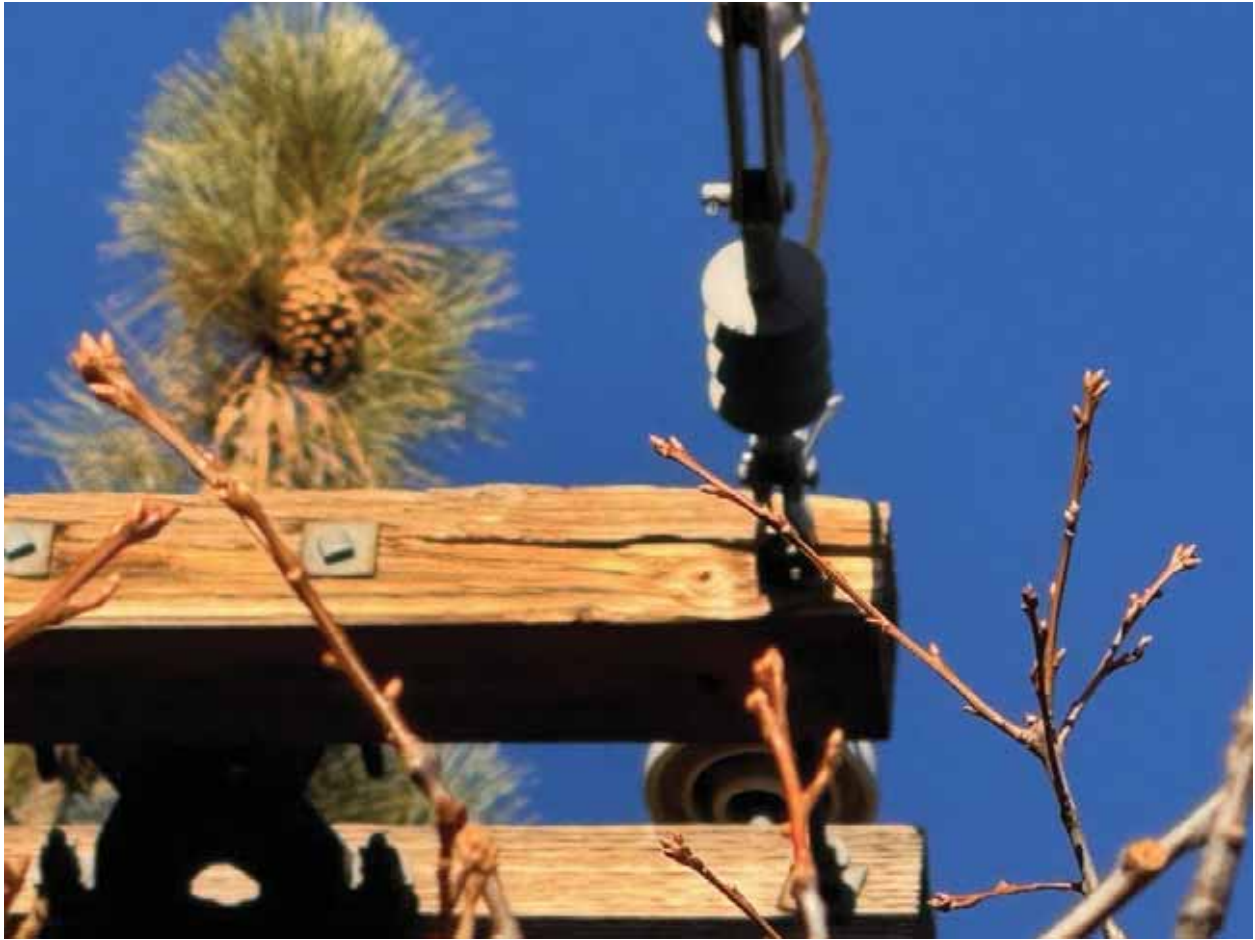
Figure 43 - Item #12 P233567 Damaged Crossarm
