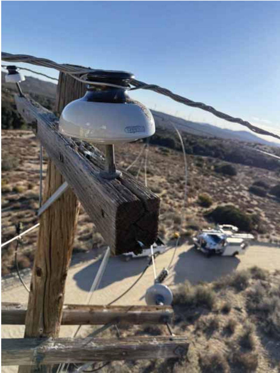
Figure 42 - Item #11 P46239 Damaged Crossarm
