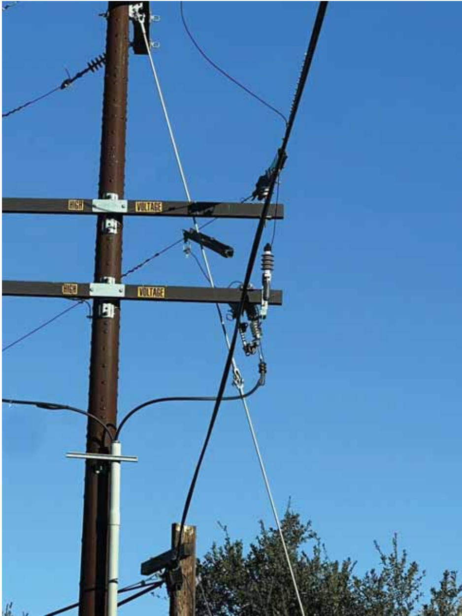
Figure 38 - Item #7 P517803 Loose Avian Protection
