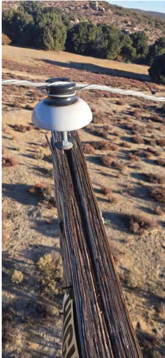
Figure 41 - Item #10 P46312 Damaged Crossarm
