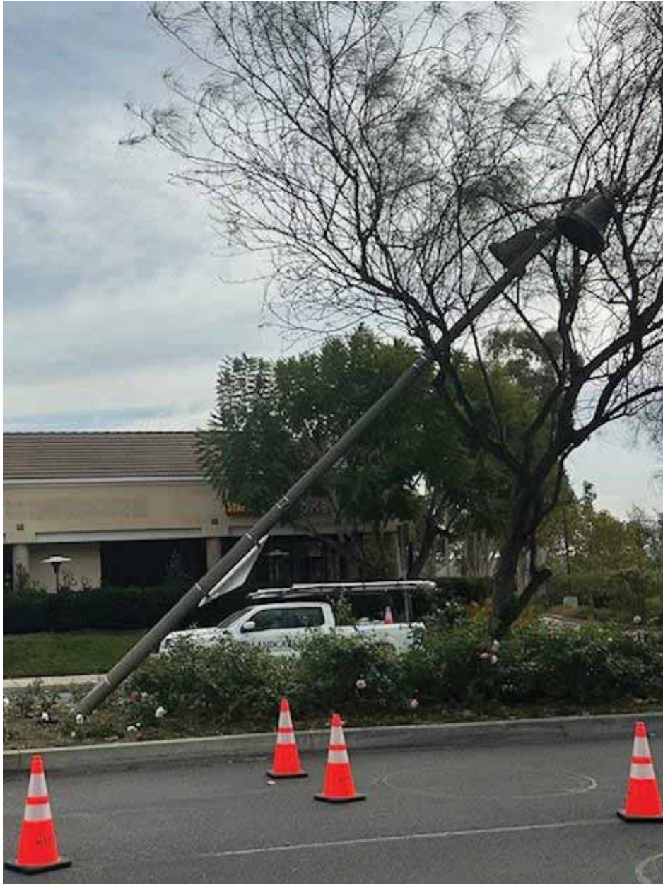
Figure 35 - Item #4 L121150 Streetlight Pole Fell Over
