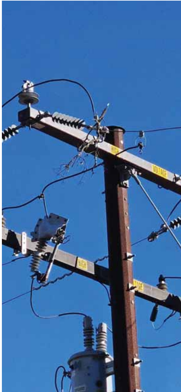
Figure 39 - Item #8 P711218 Tree Branch on Line
