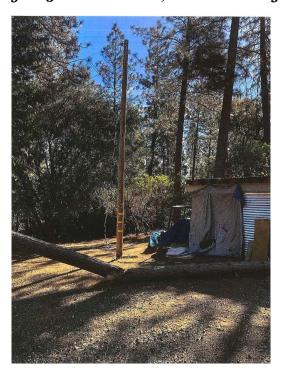
Figure 7: Tree failed and brought down conductor
