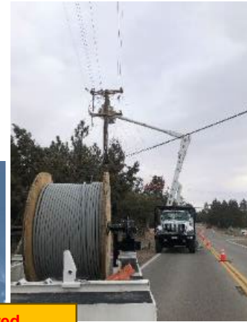
Covered Conductors
