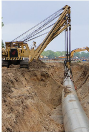
Figure 21: Replacing ten segments of pipe.
