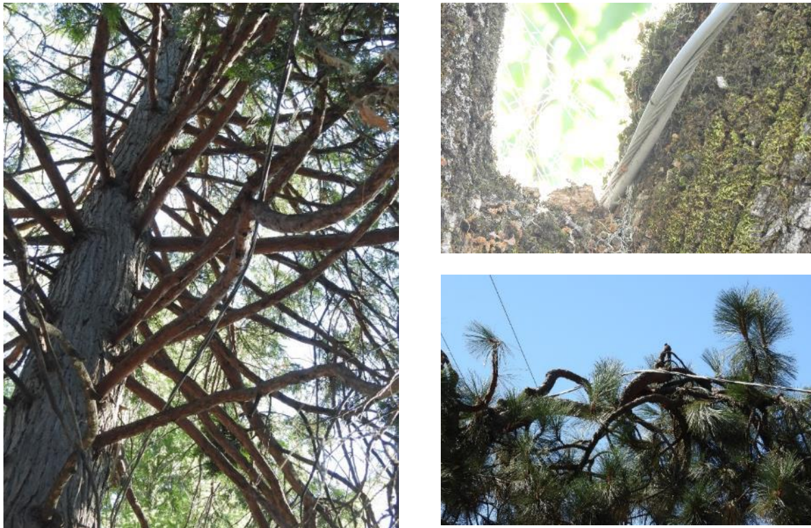
Figure 18: Photos of vegetation causing strain or abrasion taken from the ground. Photos of this condition were not captured in PG&E aerial inspection photographs.
